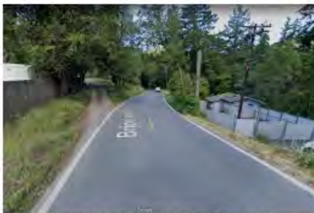
Figure 5. Photo of RCSD lift station with narrow road segment.
