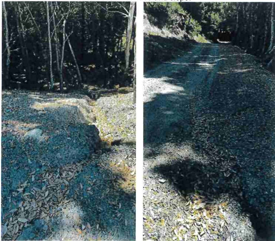
Picture 8: Road Point 14, the Discharger will out-slope the road around the base of the cultivation site fill slope to the armored fill/rocked ford at Road Point 3 and resurface the road with road rock.
