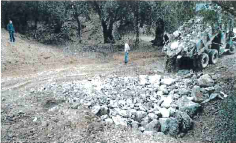
FIGURE 121D. Well graded rock armor is then backfilled into the structure and spread across the breadth of the U-shaped stream crossing, and about one-third the way up the roadbed, so that streamflow will only flow over or come in contact with resistant armor material. The armor must be spread and compacted across the design width of the expected flood flow channel width so peak flows will not flank the armored structure.
