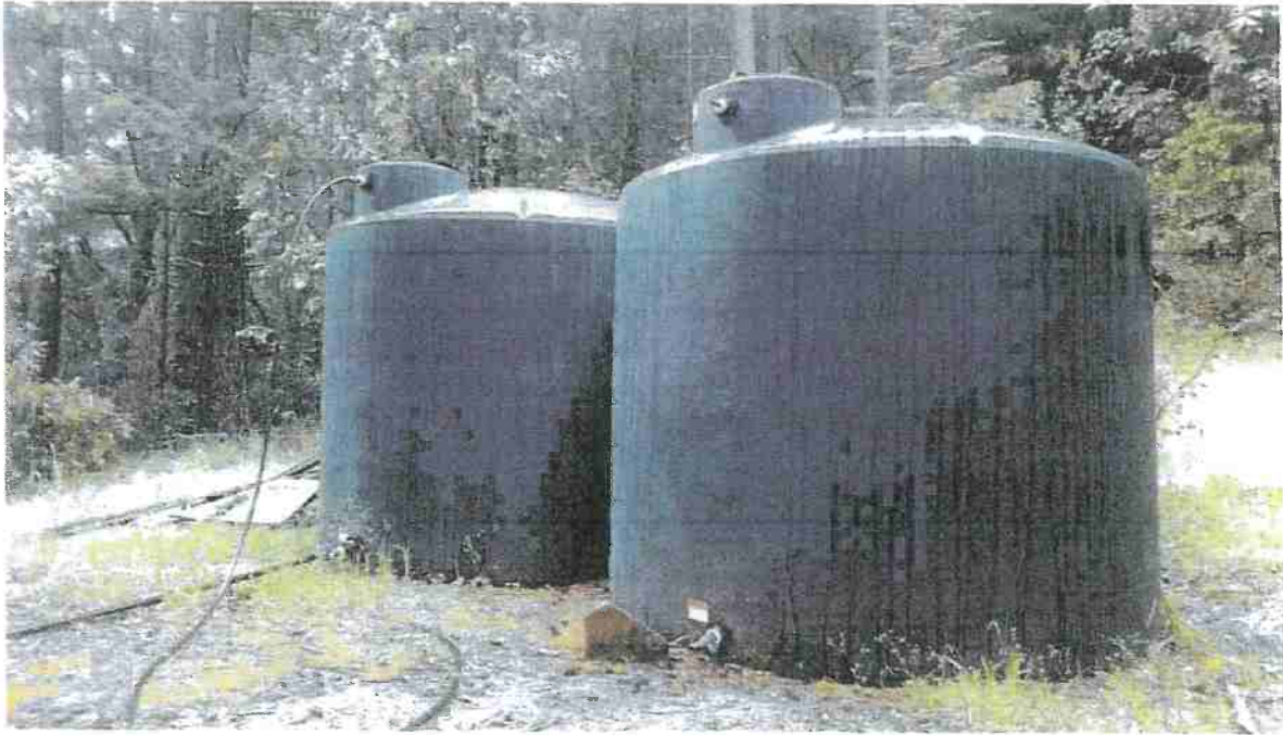
Picture 2: Two 2,500-gallon hard plastic storage tanks. Photo date 5-16-2017.
