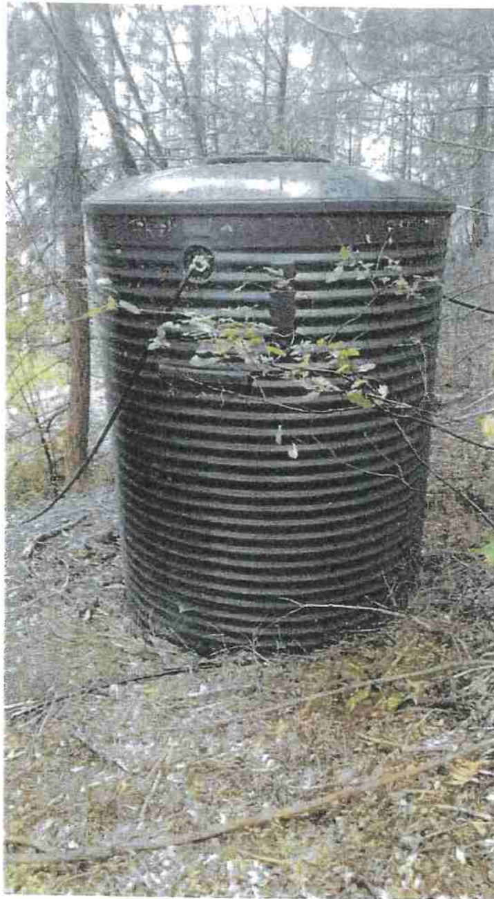
Picture 3: 1,300-gallon hard plastic water storage tanks. Photo date 5-16-2017.
