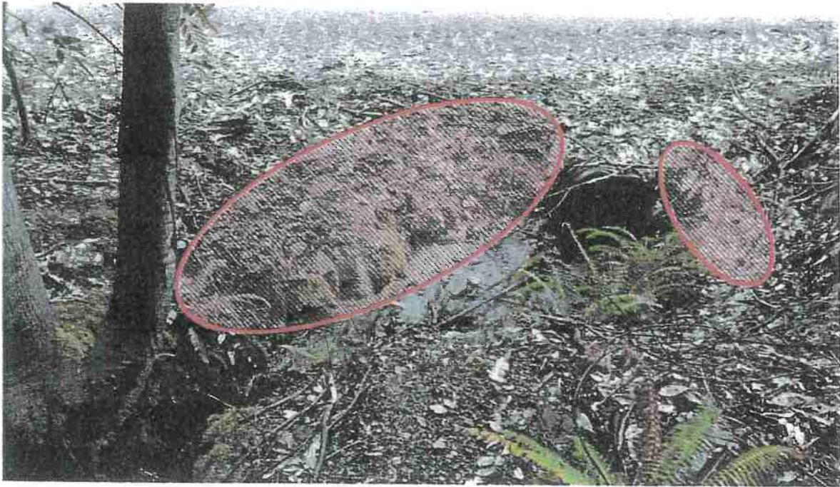
Picture 17: Crossing #3 outlet. The fill at inlet is to be regraded and rock armored. Photo date 5-16-2017.
