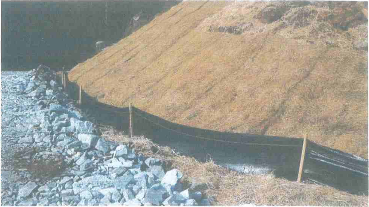
Erosion Control Matting & Silt Fencing
