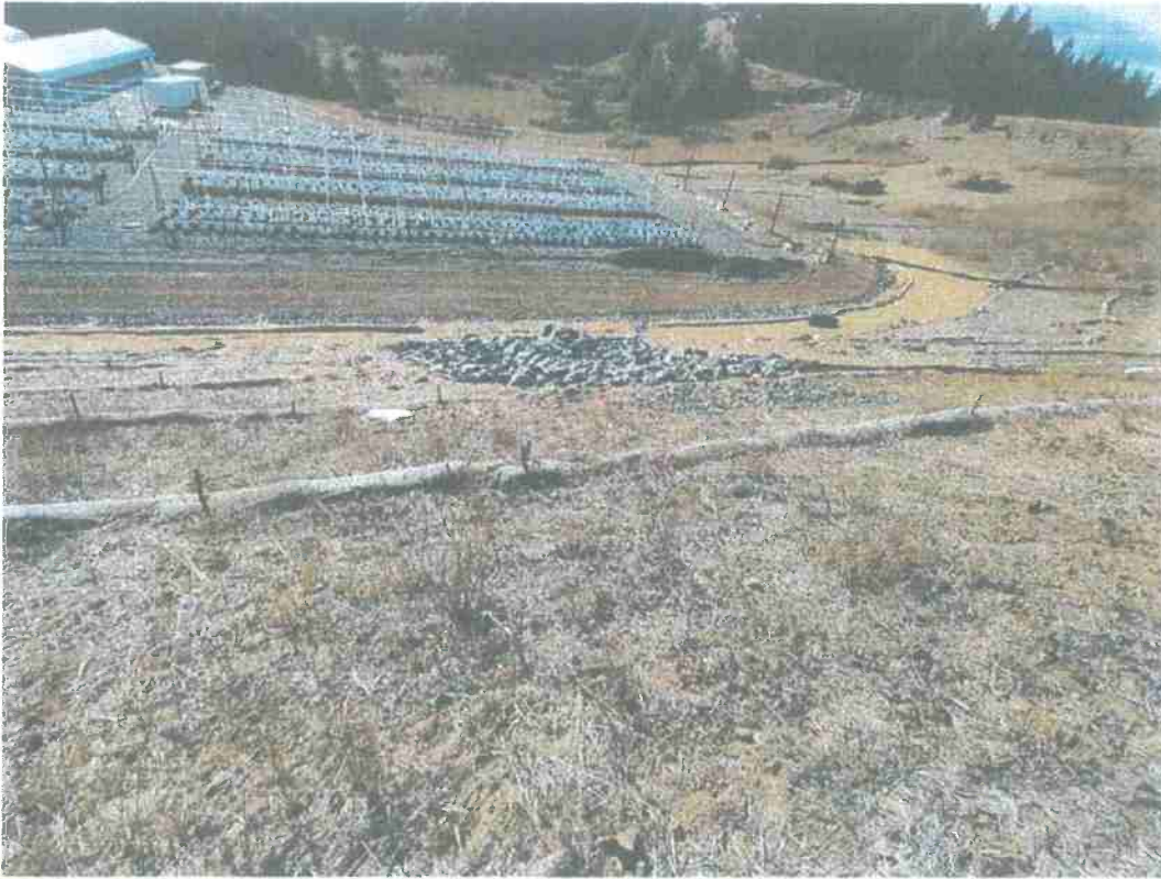
Rock buttressing installed on previously slumping cutbank
