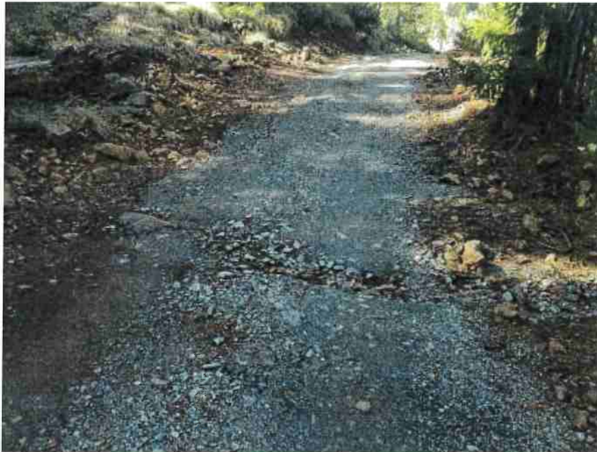
Existing ford, still functional
