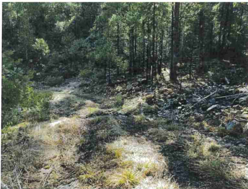
Minor erosion of roadbed but naturally rocky substrate maintains stability
