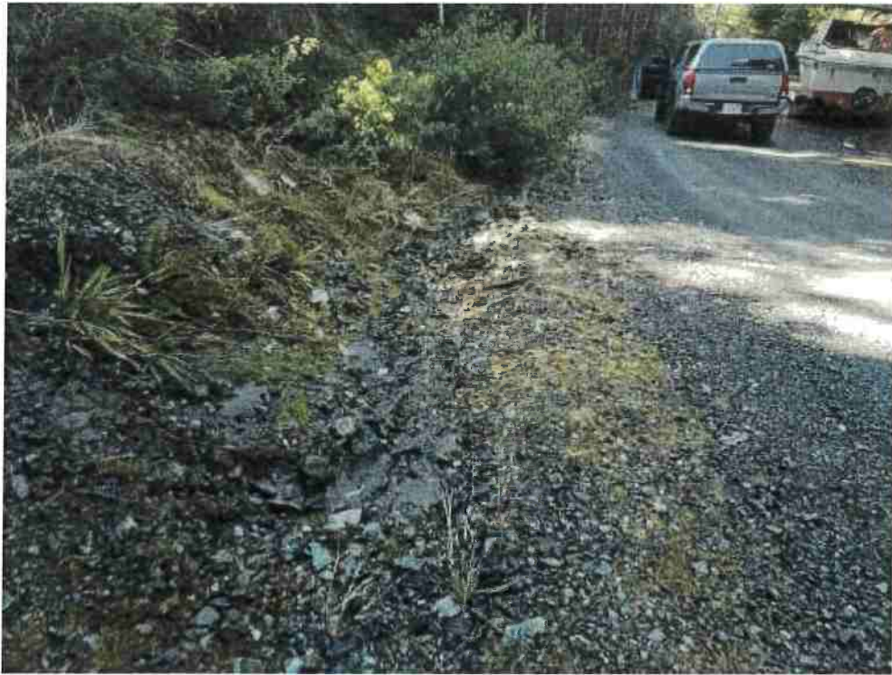
Sediment deposition in inboard ditch that diverts flow at MP20
