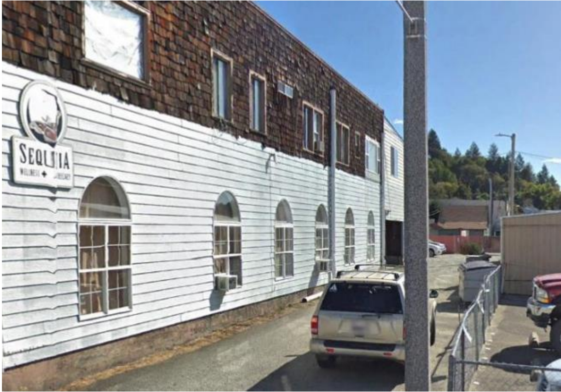
Figure 10: View of Alley & Gate from Maple Lane
