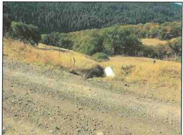
Photo #42 Ridge Rd Looking @ 18" Culvert Out
