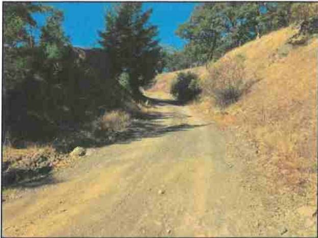
Photo #51 Ridge Rd @ Turnout Looking NW @ Curve
