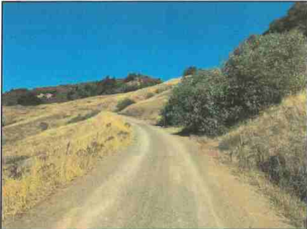
Photo #45 Ridge Rd @ Turnout Looking NW @ Curve
