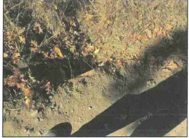
Photo #50 River Rd 12" Culvert In
