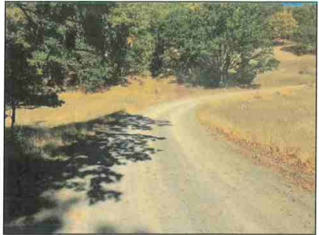
Photo #99 Ridge Rd @ Curve w/ Turnout Looking NW @ Drive
