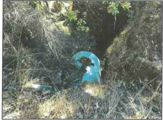
Photo #62 River Rd Looking @ 36" Culvert Out (Dual?)
