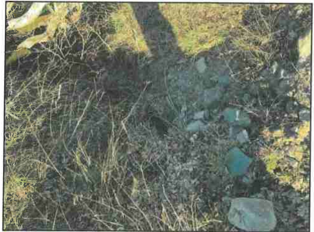
Photo #227 Intersection of Private Access Rd APN 208-241-017 Looking @ 12" Culvert In
