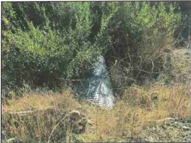
Photo #15 River Rd Looking @ 36" Culvert In
