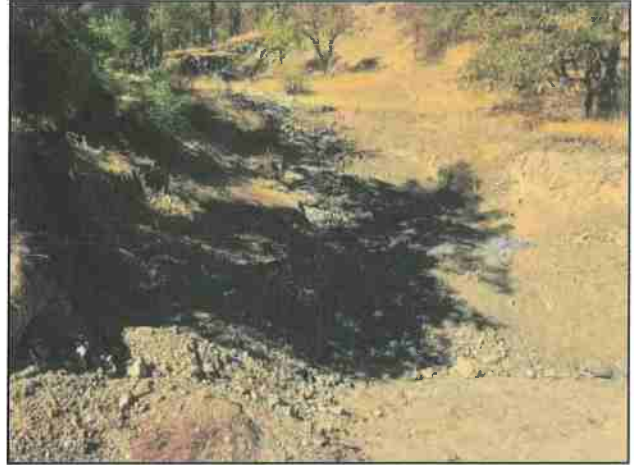
Photo #56 River Rd Looking @ Slide
