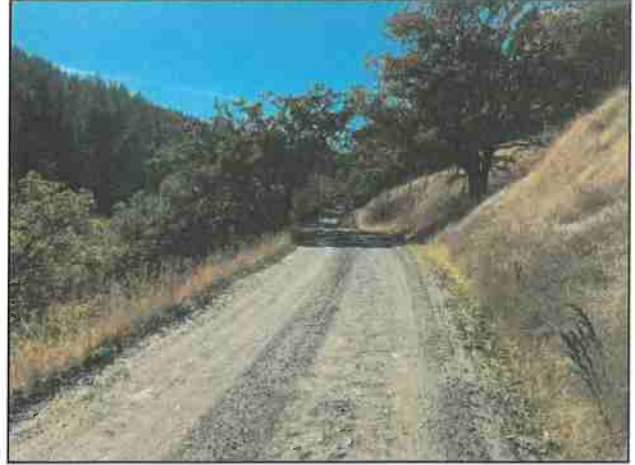
Photo #44 River Rd Looking West @ Curve w/o Turnout
