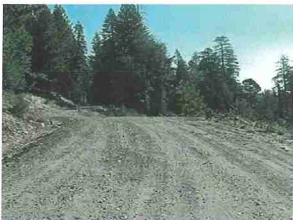
Figure 38. Pinchard Creek road immediately after project construction, 2002. Photo: Joe Hoffman, Plumas National Forest.
