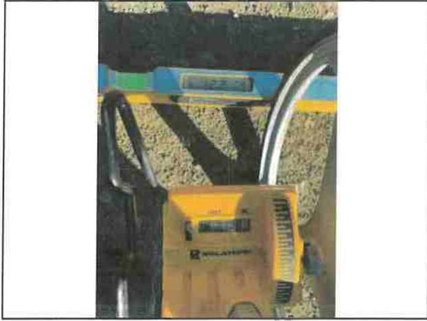
Photo #256 8 Mile Ridge Rd Width 13'6" Slope 12.2%
