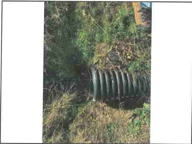
Photo #226 Intersection of Private Access Rd APN 208-241-017 Looking @ 12" Culvert Out
