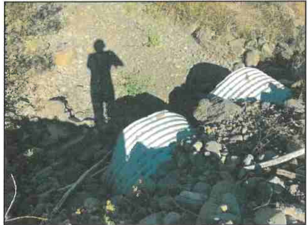
Photo #16 River Rd Looking @ Dual 36" Culverts Out
