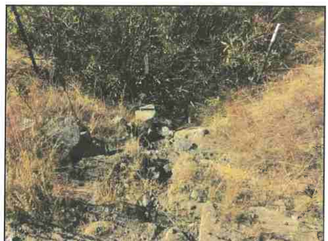
Photo #36 Ridge Rd Looking @ Culvert Out (Size-Unknown)
