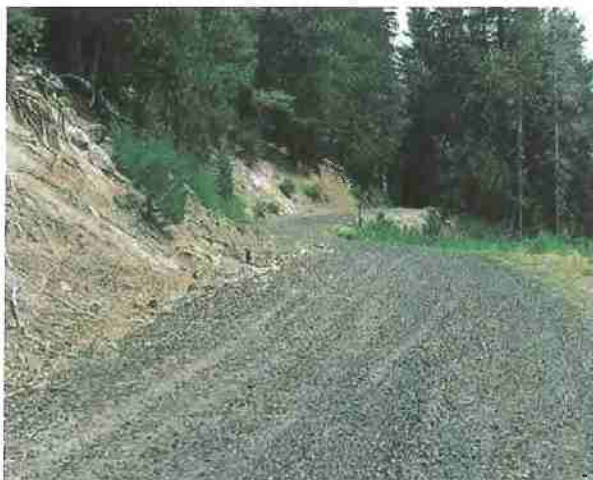
Figure 39. Pinchard Creek road two years after project construction, 2004. Note that the road surface remains in good shape without additional maintenance. Photo: Joe Hoffman, Plumas National Forest.
