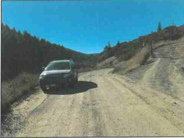
Photo #37 River Rd Looking West @ Curve w/ Pullout
