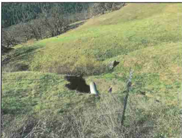
Photo #260 8 Mile Ridge Rd Looking @ 12" Culvert Out.
