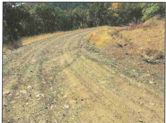
Photo #54 Ridge Rd @ Curve w/ Turnout Looking SE
