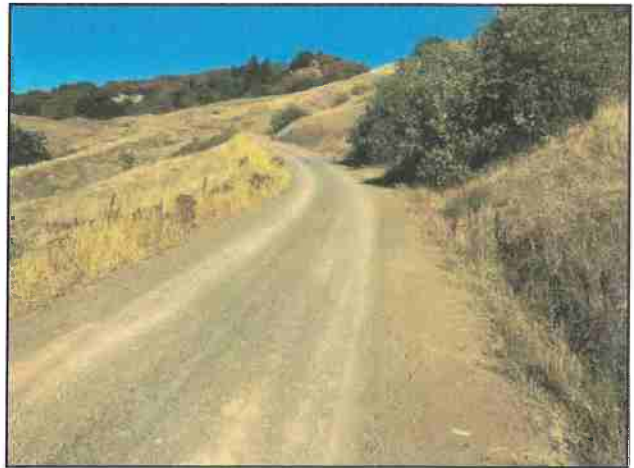
Photo #40 Ridge Rd @ Turnout Looking NW
