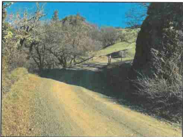
Photo #254 8 Mile Ridge Rd @ Curve w/ Pullout Looking North
