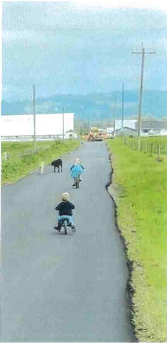
County paving road last week
