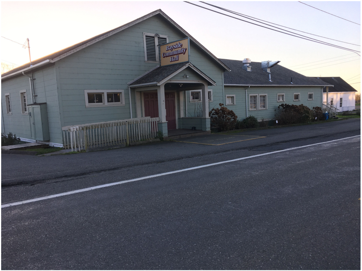
192 Community Hall, photo by the National Register of Historic Places.
