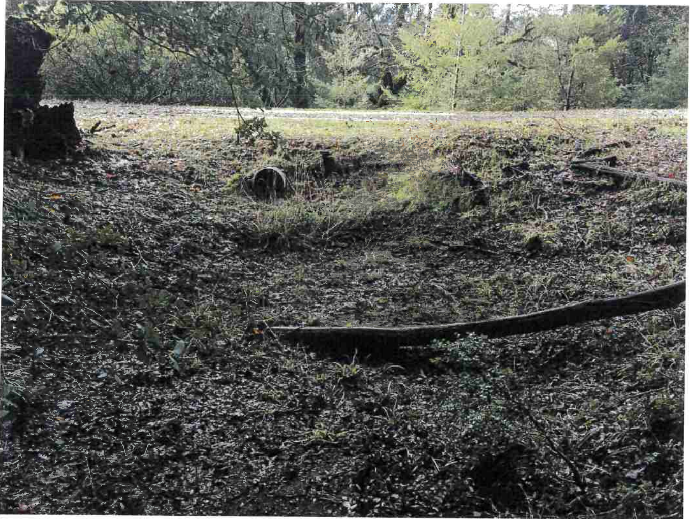
Picture 10: Inlet of Crossing #1. The small pond is in the foreground. Photo date 12-2-2016.
