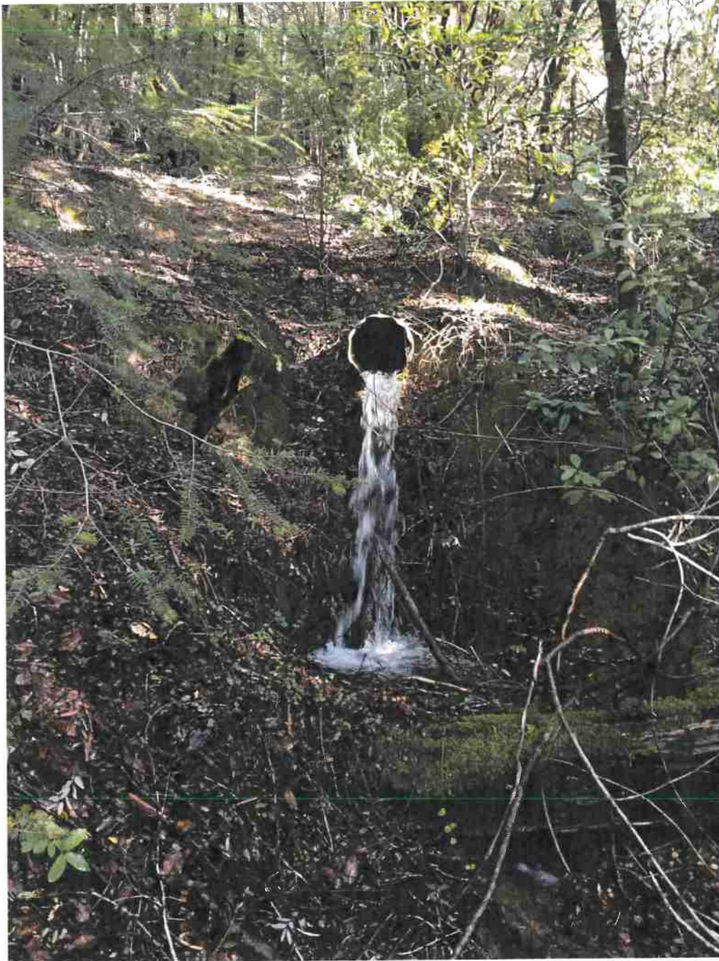
Picture 17: Crossing #5 outlet. Photo date 12-16-2016.
