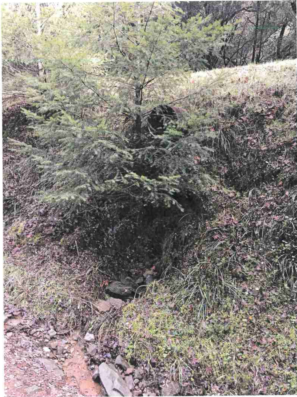
Picture 11: Outlet of Crossing #1. The Applicant shall rock armor the outlet from the small Douglas-fir tree down to the inside ditch. Photo date 12-2-2016.
