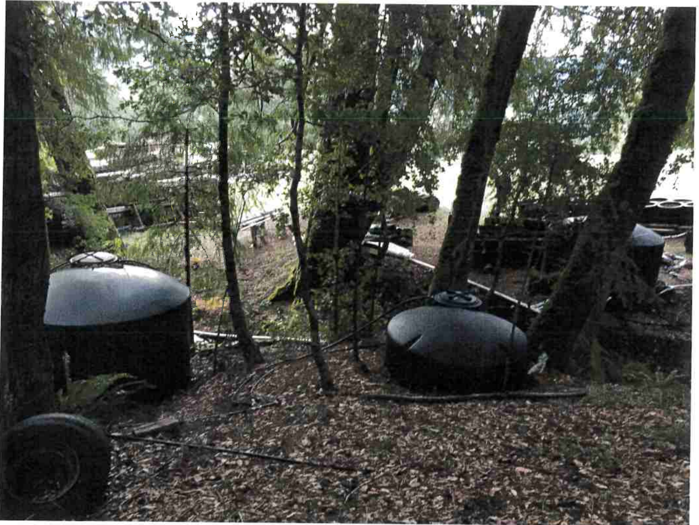
Picture 23: 2,500, 1,550, and 500 gallon water tanks clustered near the Class III stream channel. CDFW recommends that the Applicant shall remove all tanks, diversion infrastructure, and any other stored material located directly adjacent to the stream channel, and relocate outside of the SMA, or as far away from the stream channel as possible. Photo date 12-2-2016.
