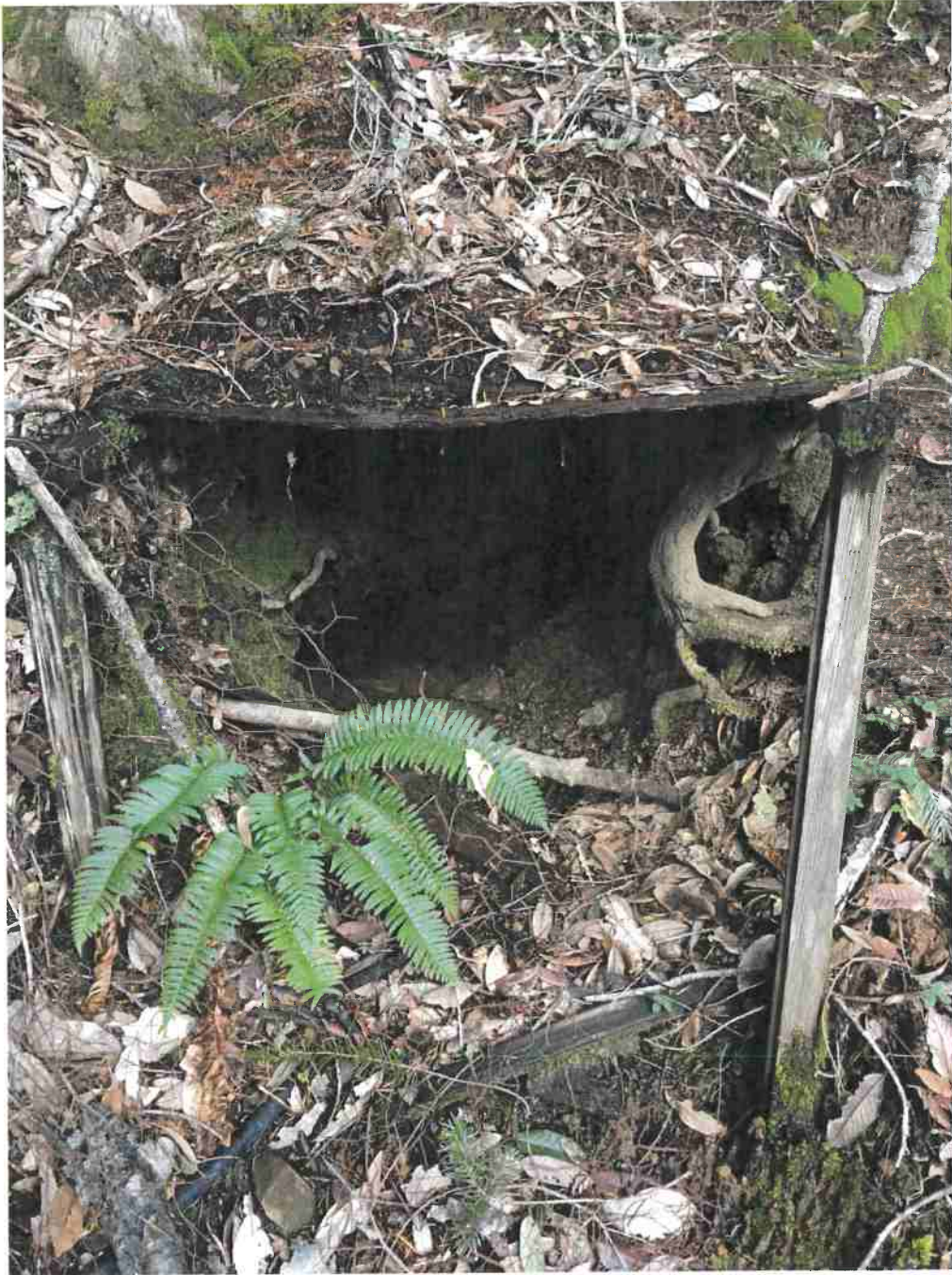
Picture 7: POD #3. Photo date 12-2-2016.
