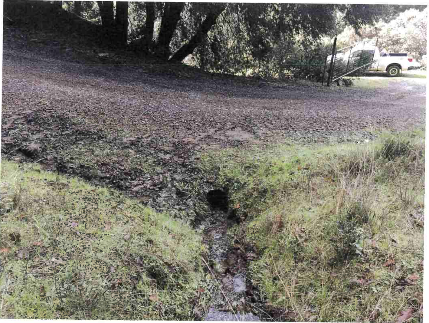
Picture 12: Inlet of Crossing #2. Photo date 12-2-2016.
