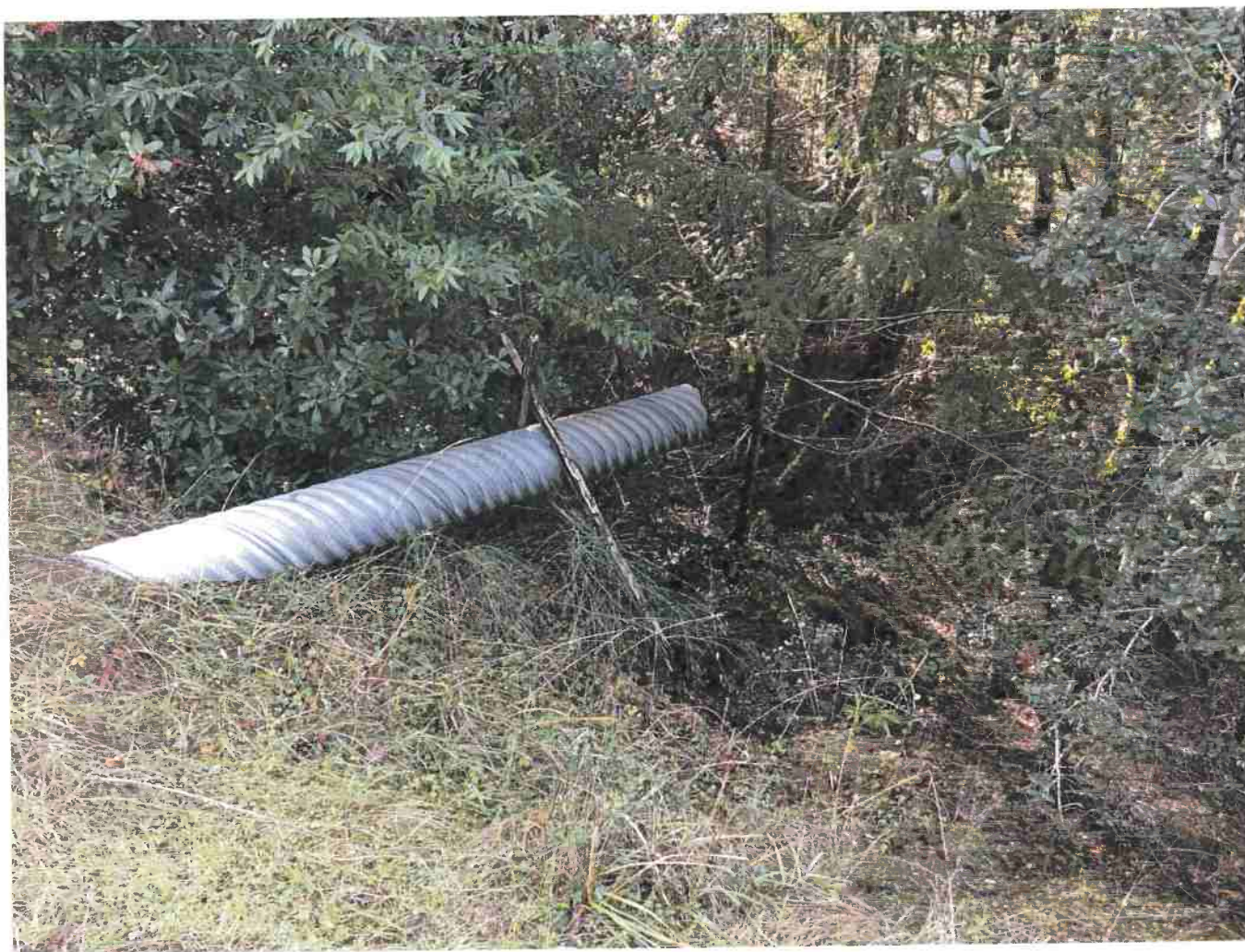
Picture 19: Crossing #6 outlet. Photo date 12-16-2016.
