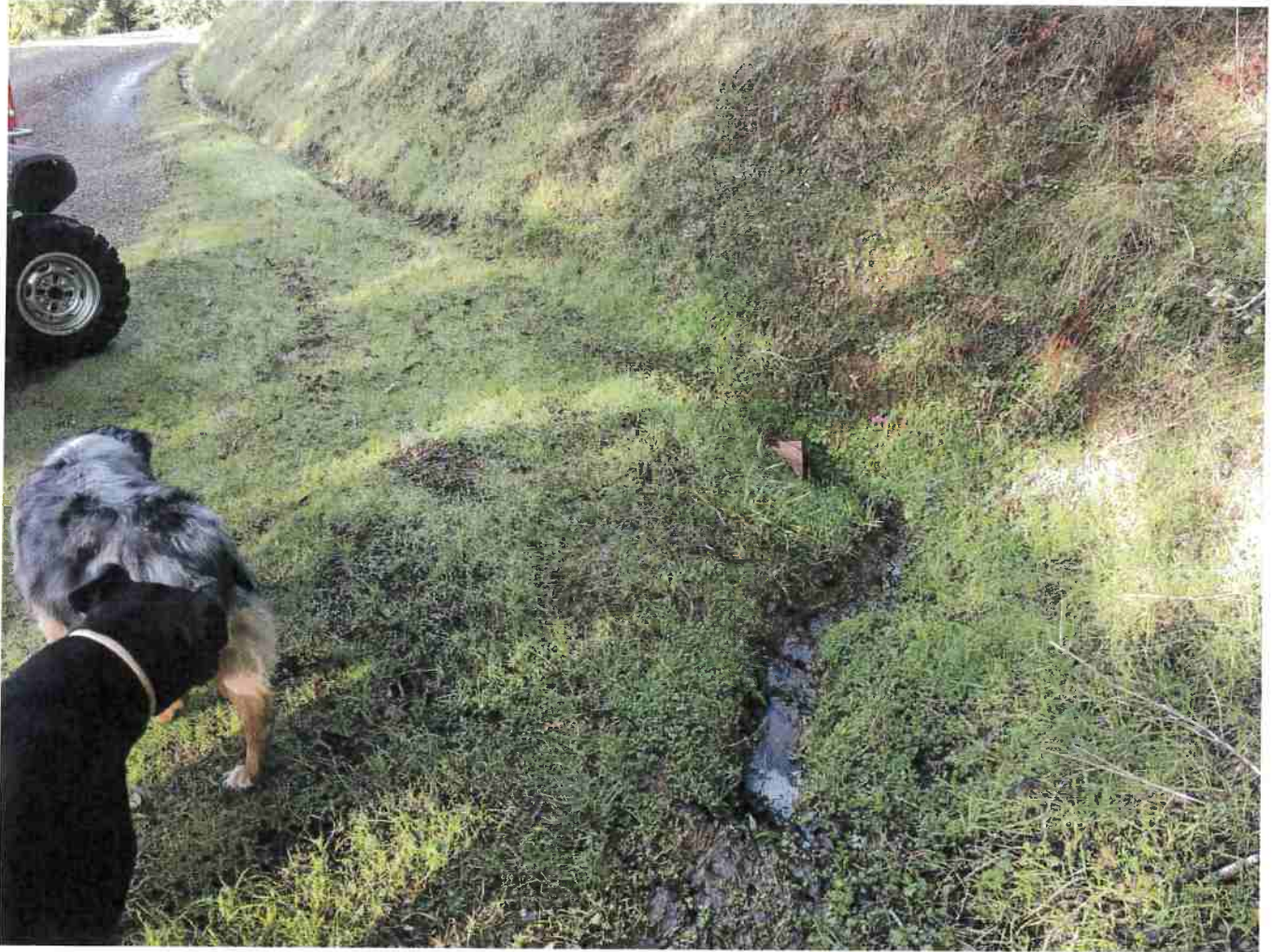
Picture 20: Inlet of Crossing #6. Photo date 8-31-2016.
