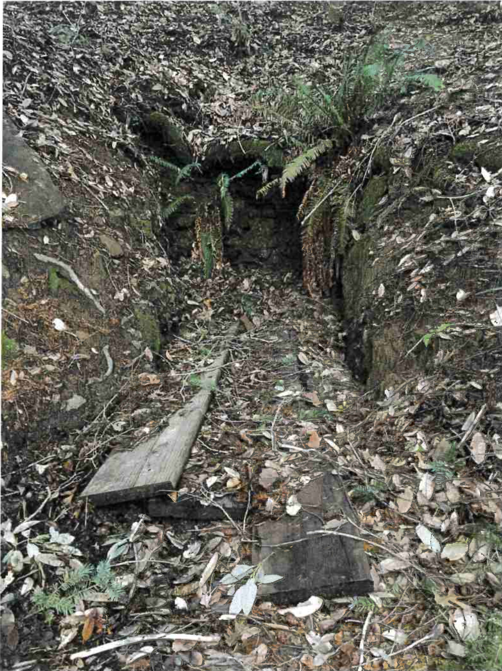
Picture 4: POD #2. During the CDFW consultation, the Applicant agreed to discontinue the use of this diversion and remove all associated infrastructure. Photo date 12-2-2016.
