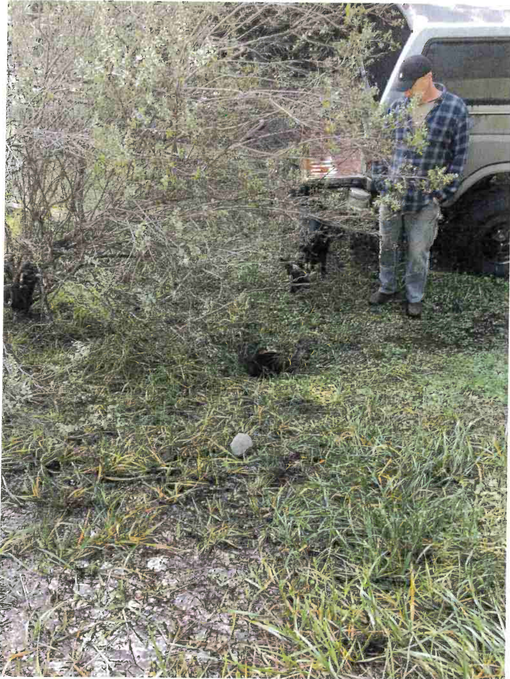
Picture 21: Inlet of Crossing #7. Photo date 8-31-2016.
