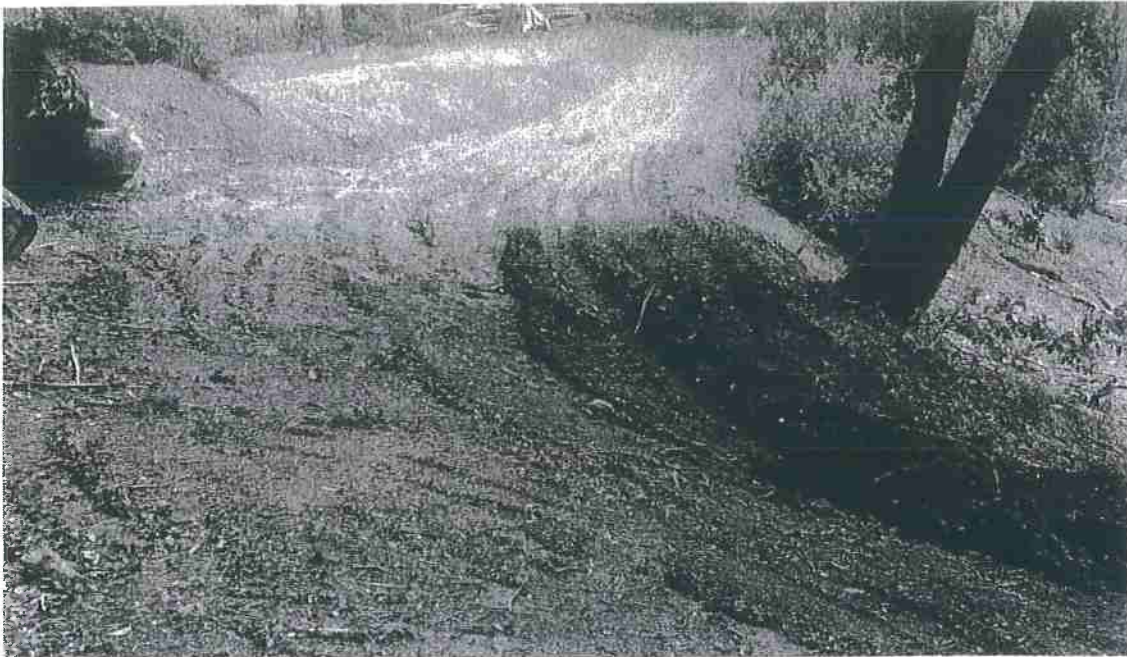
Site 19 looking up grade towards Site 18. Note rutting, concentrated road surface runoff, and the disturbed area/removed cultivation area, to the upper left. Also, in the photo that is difficult to discern is the cultivation-related soils and perlite on the road surface and removed cultivation area.
