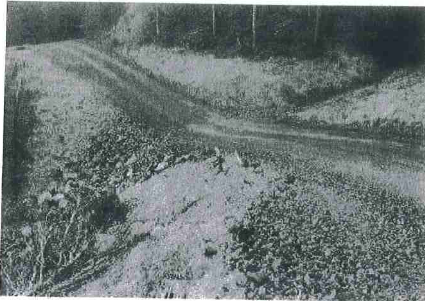
FIGURE 120. This armored fill crossing of a steep, ephemeral stream was constructed to provide a low maintenance crossing. The crossing has been deeply dipped to reduce the volume of road fill and to eliminate the potential for stream diversion. The fill slope has been heavily armored through the axis of the crossing to contain flood flows and prevent down-cutting. Armored fills cannot be used on fish bearing streams.
