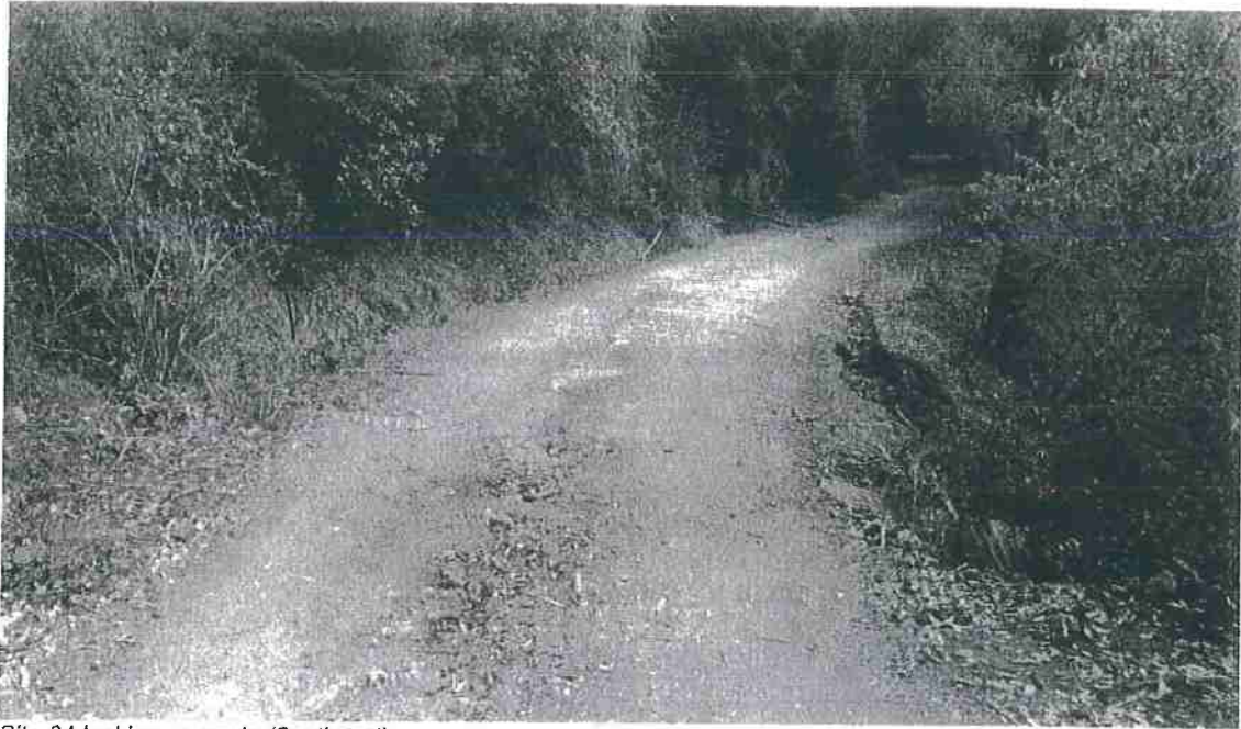
Site 01 looking up grade (Southeast).
