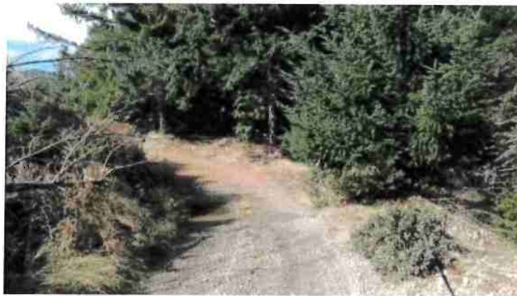
Figure 5. Road Point 7, outslope for proper drainage.
