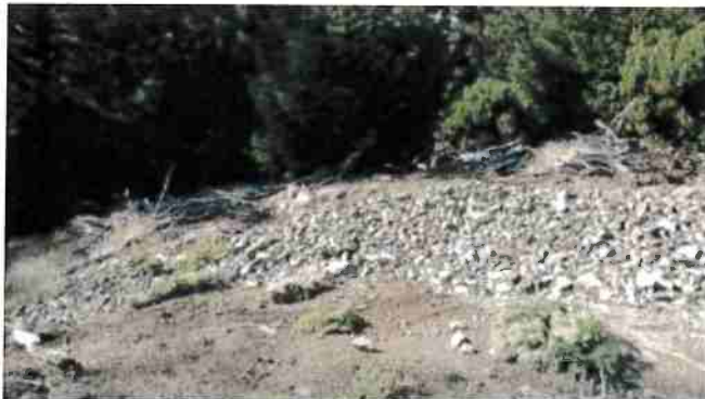
Figure 19. Rocked drainage outlet for site D.
