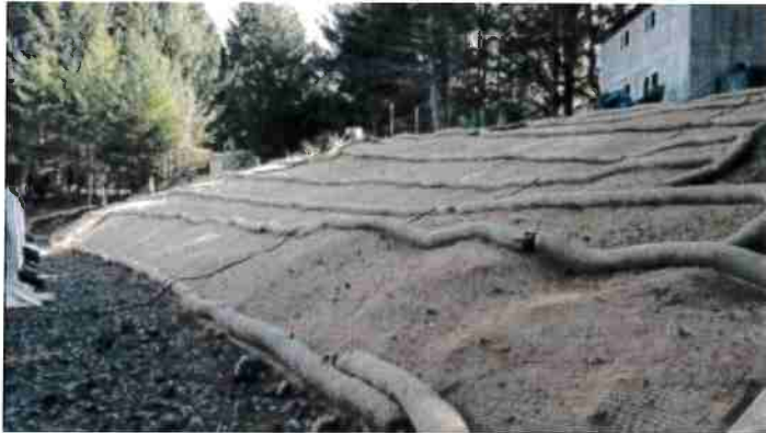
Figure12. Erosion control mat on cutbank between the greenhouse and the house site
