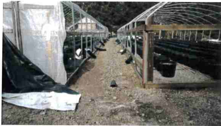
Figure 3. Rocked drain between the upper set of greenhouses, drains to the north.
