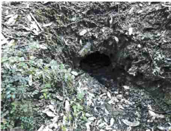
Photo #174, location 44 north 18" cmp inlet
