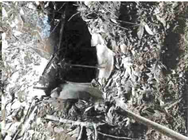
Photo #222, location 55 south side of road 18" cmp inlet.
