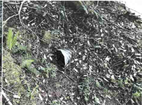
Photo #195, location 49 Inorth end 18" cmp inlet.
