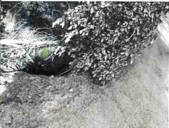
Photo #210, location 51 north side road 18" cmp inlet.
