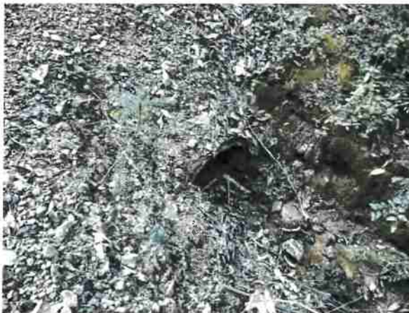
Photo #162, location 41 south end of 18" cpp outlet.
