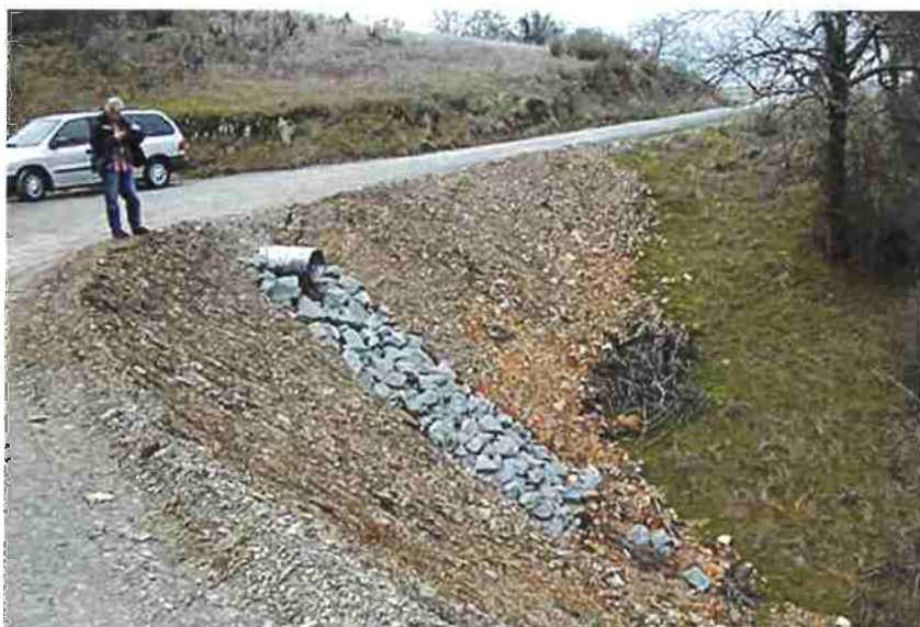
Figure 25. Eroding fill slope and culvert failure due to plugging at inlet and diversion of flow across the road. Photo: Bill Weaver, Pacific Watershed Associates.
