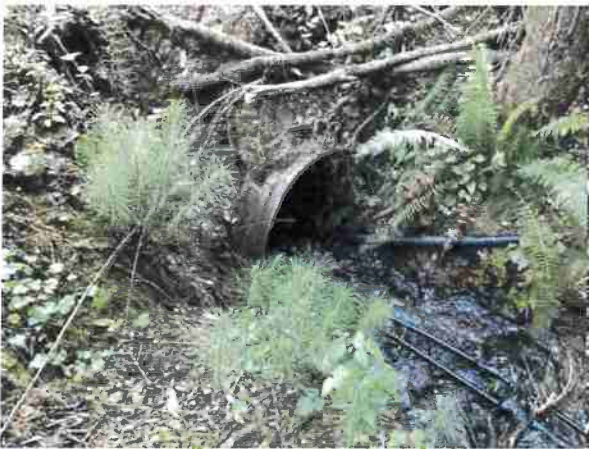
Photo #184, location 45 south east side of road near 18" cmp inlet.
