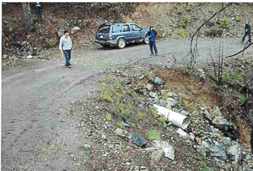
Figure 25. Eroding fill slope and culvert failure due to plugging at inlet and diversion of flow across the road. Photo: Bill Weaver, Pacific Watershed Associates.
