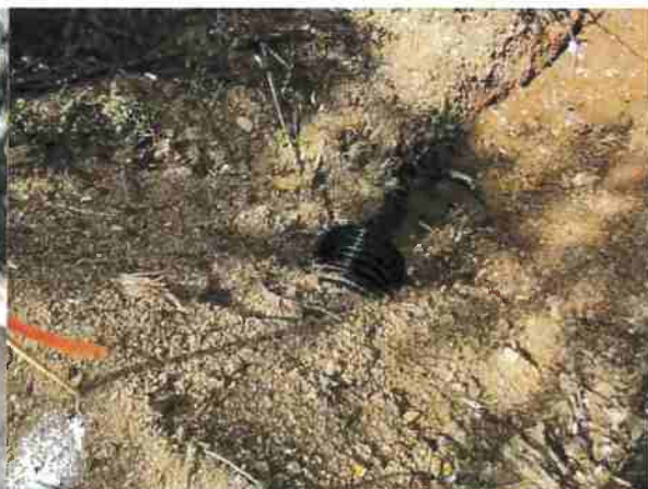
Photo #145, location 37 south side road 18" cpp outlet.
