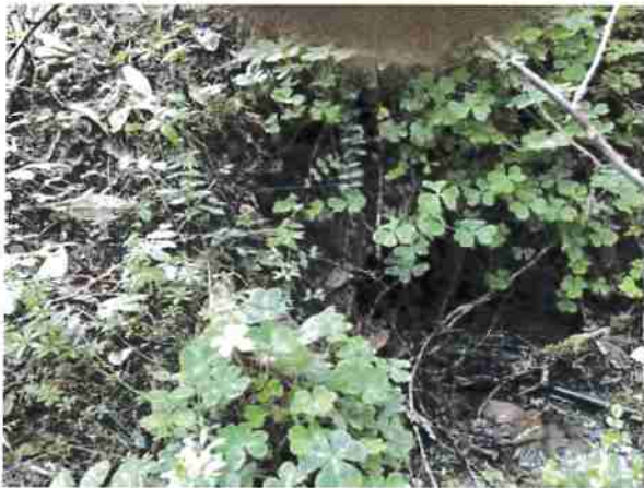
Photo #209, location 51 south side road 18" cmp outlet.
