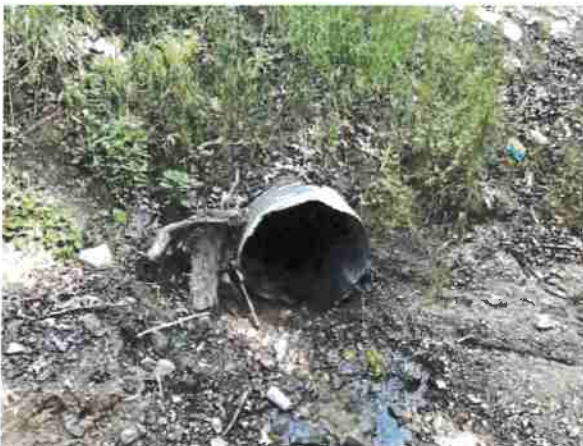
Photo #275, location 69 west end of 30" cmp outlet.
