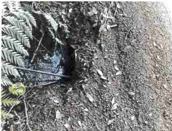
Photo #203, location 50 south side of road 18" cmp inlet.
