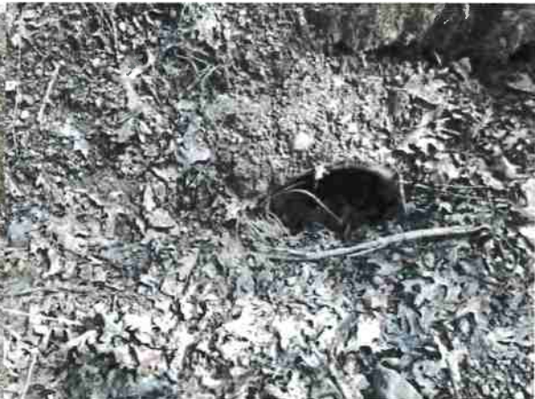
Photo #276, location 69 east end of 30" cmp inlet.
