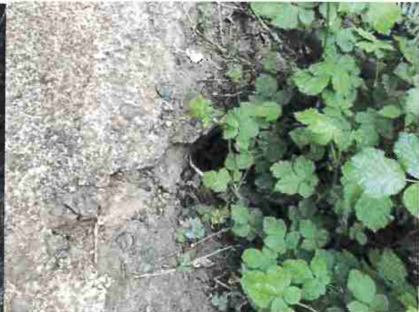
Photo #161, location 41 north end of 18" cpp Inlet.
