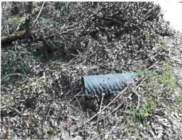
Photo #196, location 49 south end 18" cmp outlet.
