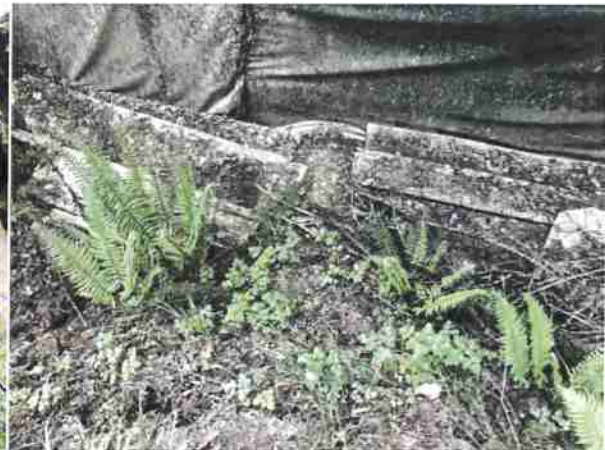
Photo #171, location 43 east 18" cmp outlet.
