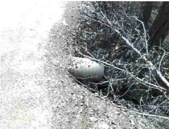
Photo #205, location 50 north side of road 18" cmp outlet.
