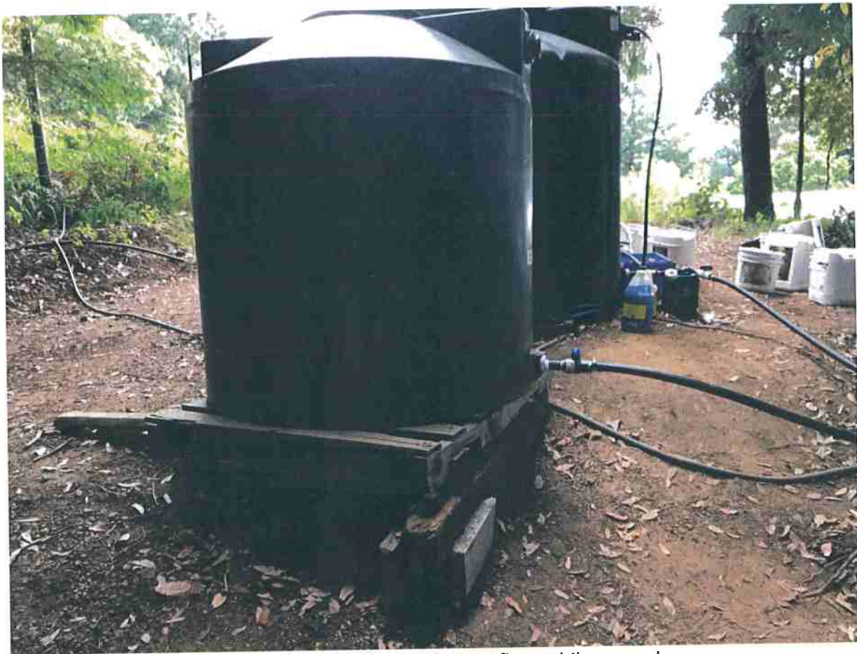
Water tanks need to be place on flat stabile ground. Completion date will be 06/30/2017
