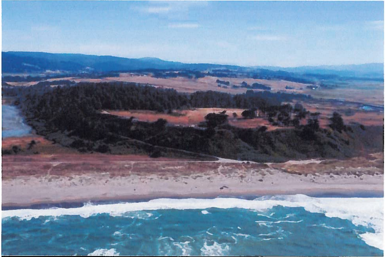
Figure 2. Oblique view of proposed action area showing treatment dunes and BLM maintained day use area to rear of dunes at the base of Table Bluff. Copyright © 2002-2015 Kenneth & Gabrielle Adelman, California Coastal Records Project, www.californiacoastline.org
