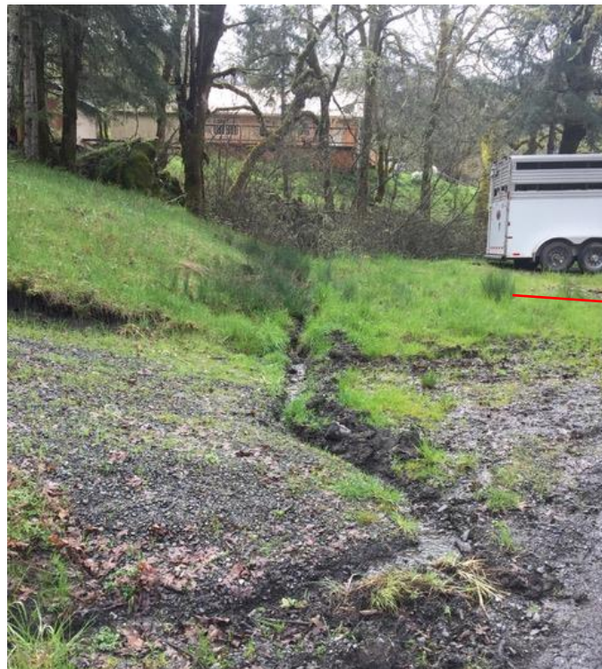
Photo 17. Road A Project 3 – future flow through culvert marked by arrow
