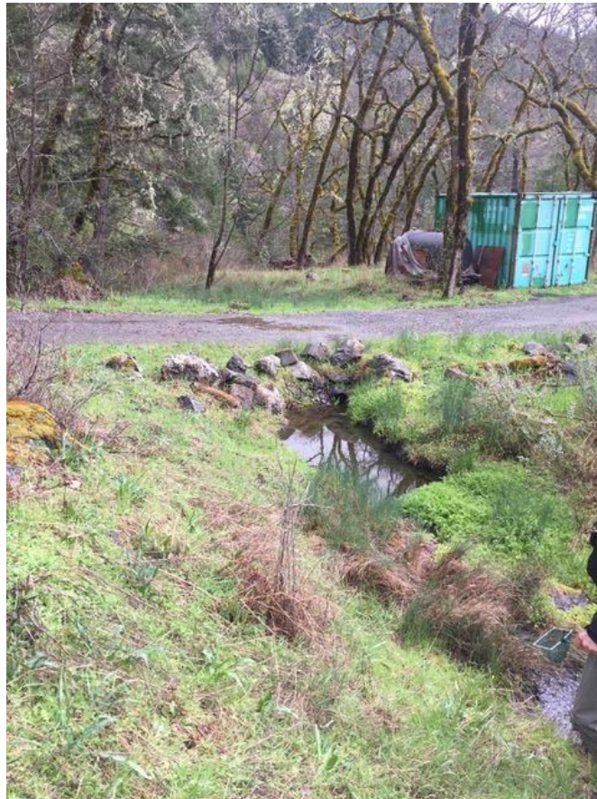
Photo 14. Project 2 on Road A – LDS at inlet
