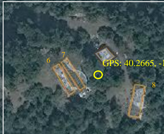
Structures - Site B.
