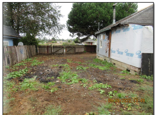
Railroad Drive after abatement
