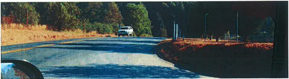
Above: 2008 picture at stop limit line on Flower-NcNeil Road at its intersection with Country Club Drive. Looking south along Country Club Drive towards Willow Creek.
