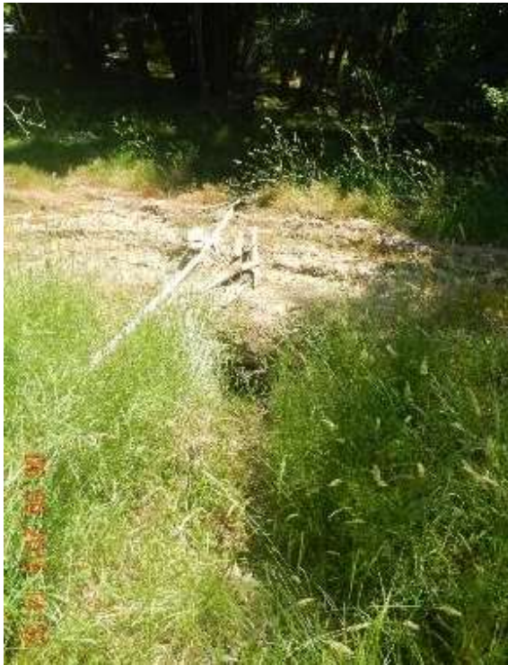
Lower reach of skid access road. The road fill and 24” culvert has been removed. Pre-restoration, left. Post restoration right.
