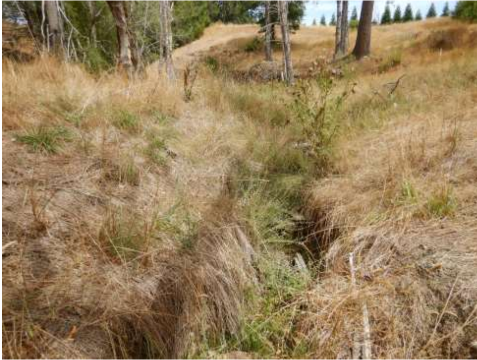
Restored stream channel showing minor incision. August 21, 2019 – Post restoration
