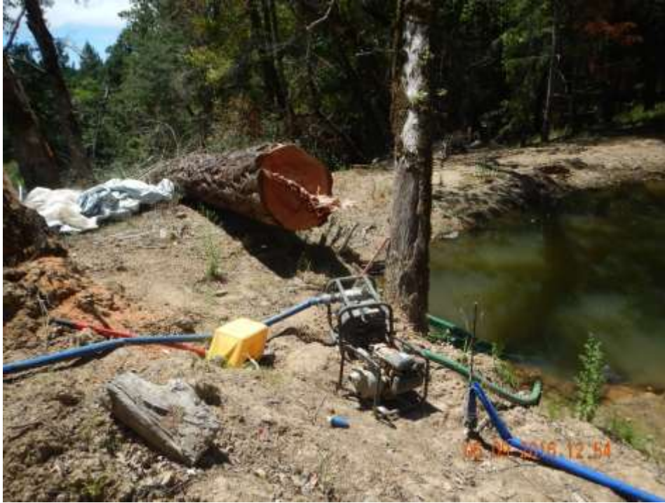
Earthen dam – pre-restoration
