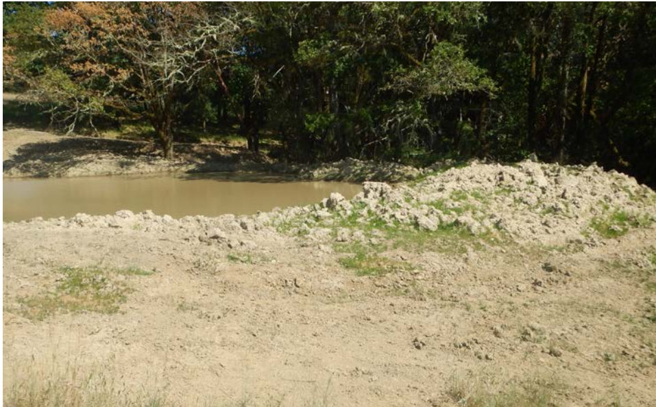
Pond looking east, showing the fillslope and berm.
