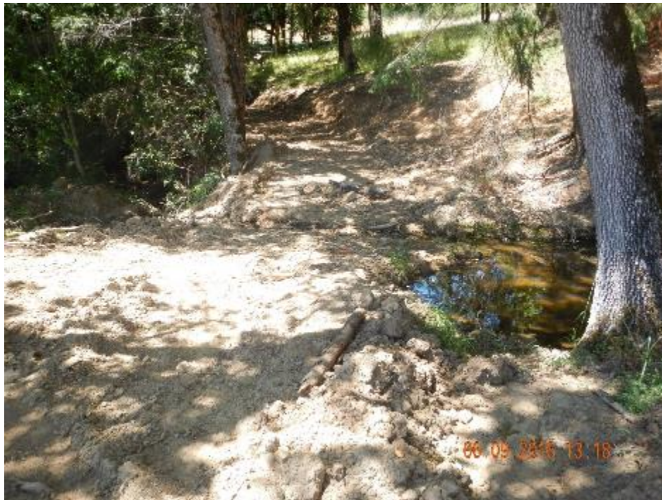
Fill crossing below the dam, looking west to the graded road.
