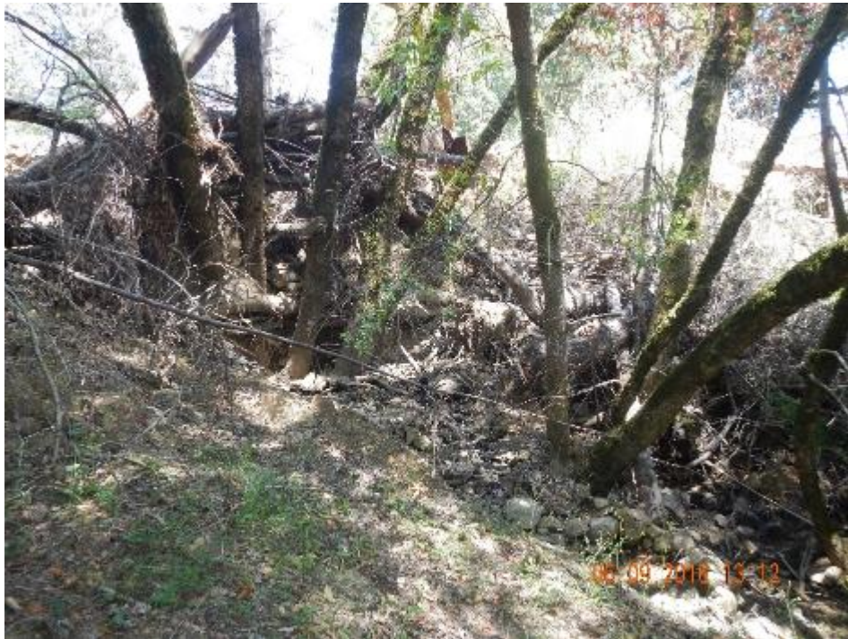
Downstream of dam fill looking up channel.
