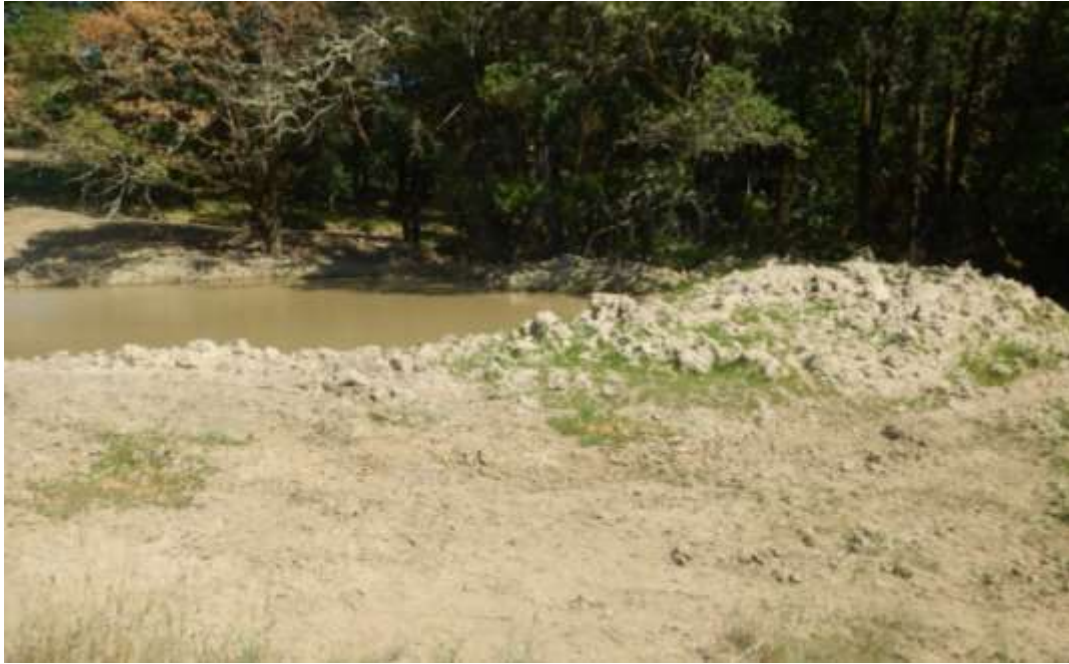
Pond looking east, showing the fillslope and berm. Pre-restoration.
