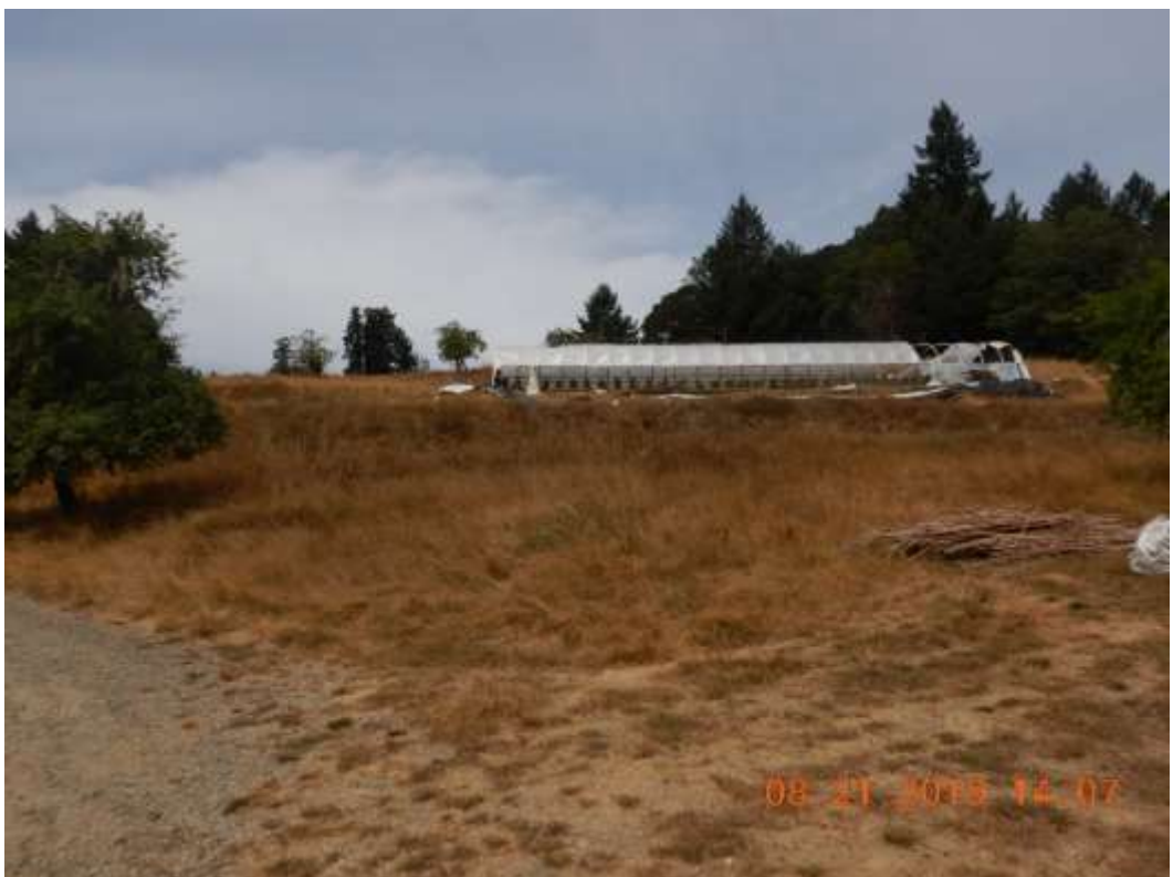
Three greenhouse flats, looking north. The flats will be regraded and contoured to original grade. August 21, 2019
