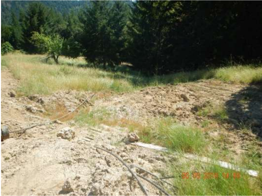
Downslope of culvert is heavily disturbed. A Class III stream channel develops below.
