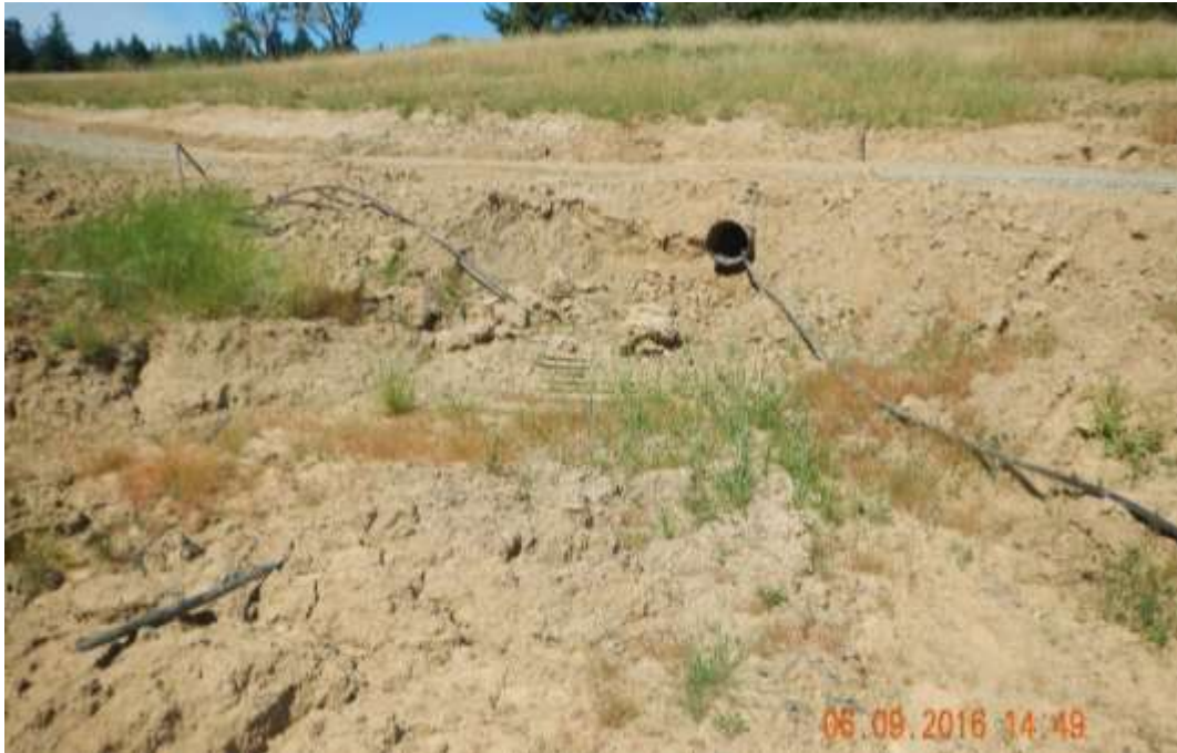
12" culvert at head of Class III stream, draining the inboard ditch and surface flow. 2016 photo.
