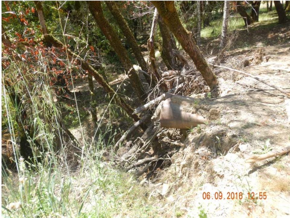
Overflow culvert for pond extending from dam fill.
