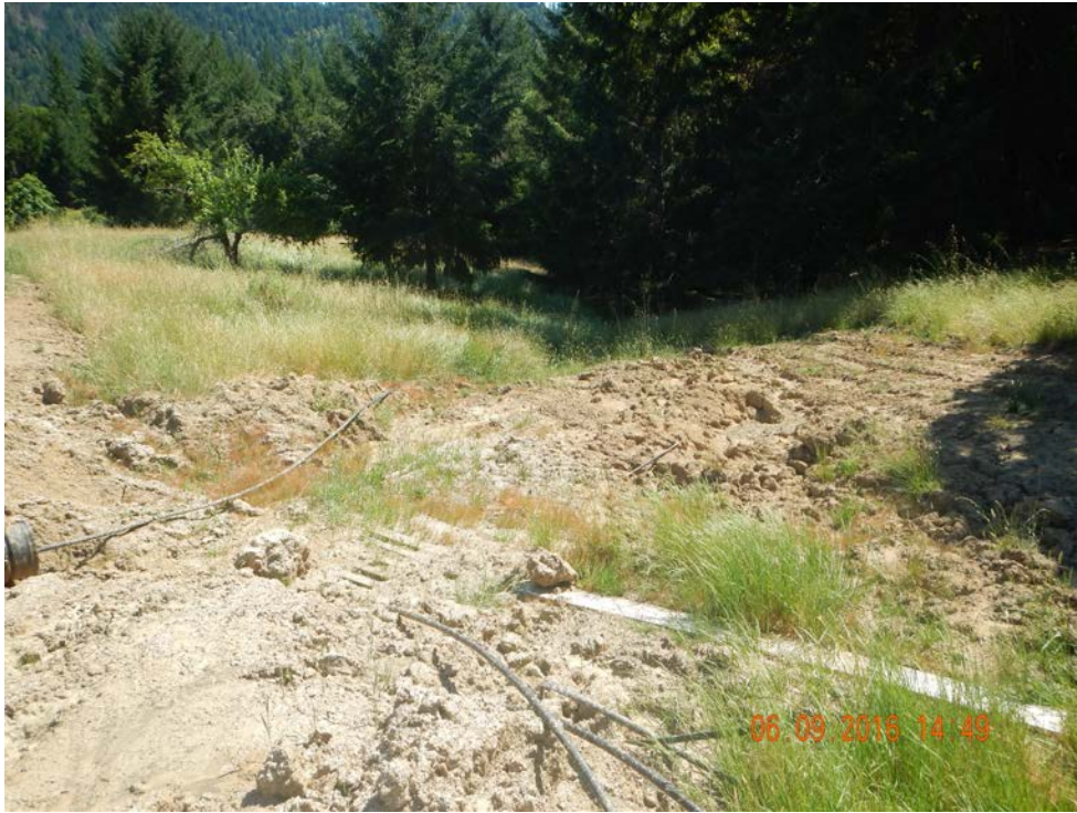
Downslope of culvert is heavily disturbed. A Class III stream channel develops below.
