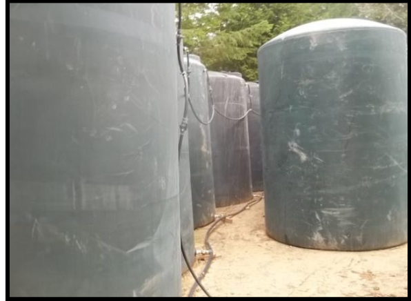
Eight (8) 5000 gallon storage tanks= 40,000 gallon storage
