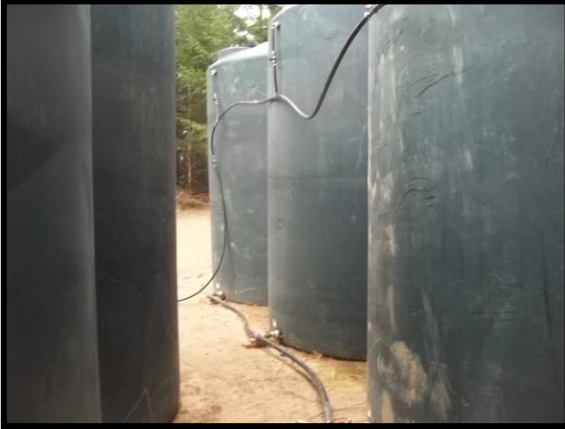
Eight (8) 5000 gallon storage tanks= 40,000 gallon storage
