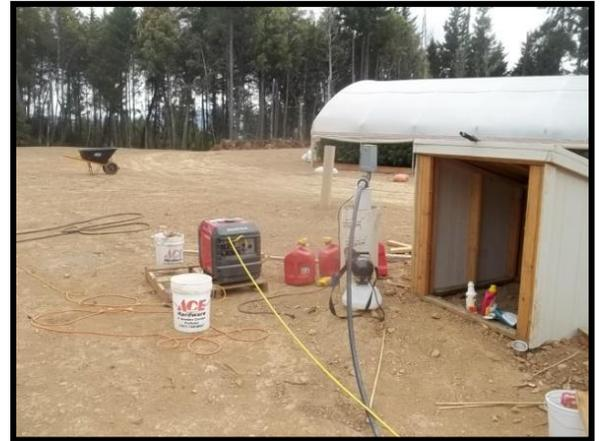
**Water is delivered to eight (8) 5000 gallon tanks (GPS 888) by a gas generator and conveyed by a 1" ADS Polyflex Potable Grade (IPS) pipe. From the storage tanks water can be directed two ways:**
