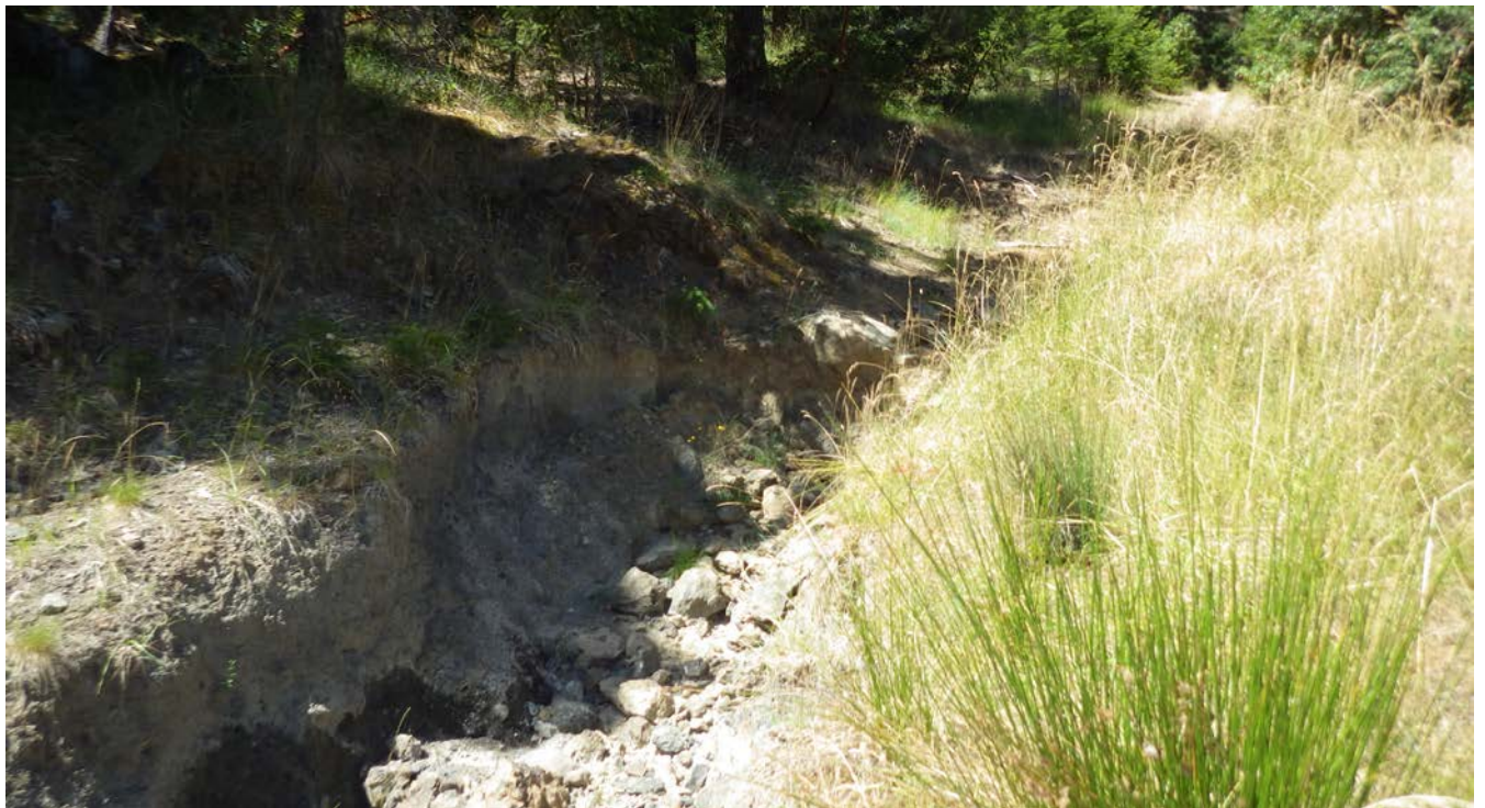
Photo 12 - Area 1– Active erosion in channel zone of Class III at the overflow channel of the pond
