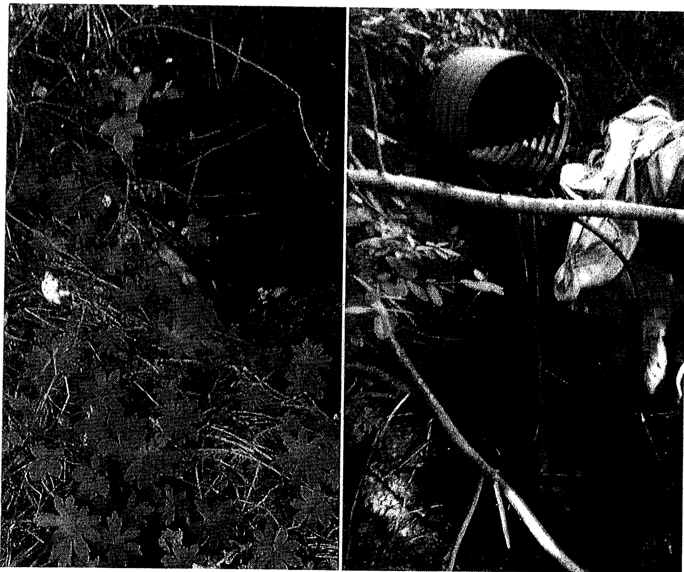
Map Point 4: These pictures show the inlet and the outlet of the existing 24-inch diameter culvert, Class II watercourse crossing at Map Point 4. This culvert is not set to grade of the watercourse and is undersized. This culvert should be replaced with a new 54-inch diameter culvert installed per the attached BMPs. Photo date 3-4-2020.
