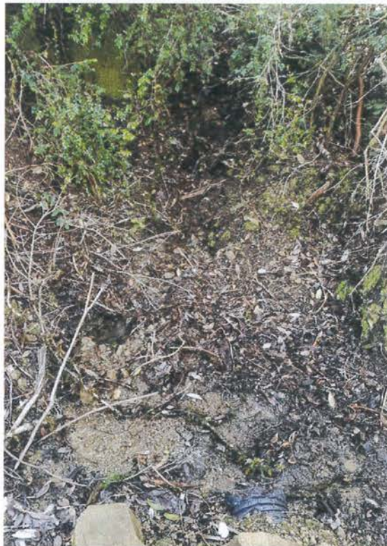
Site 58. Looking upstream of the inlet. Flows go subsurface in the duff before the inlet.
