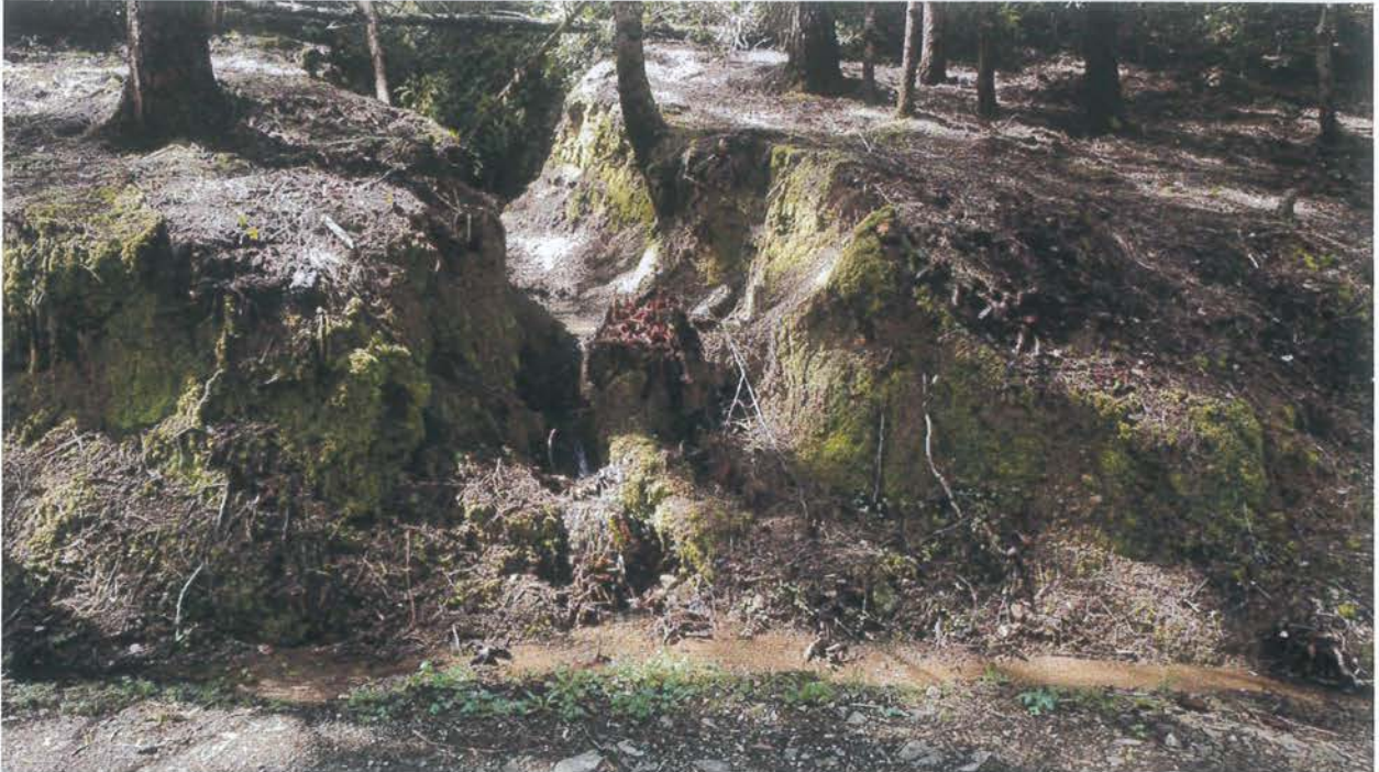
Site 51. Class III intercepts inside ditch and primarily drains to the right side of the photograph into the inlet of the crossing at Site 50.
