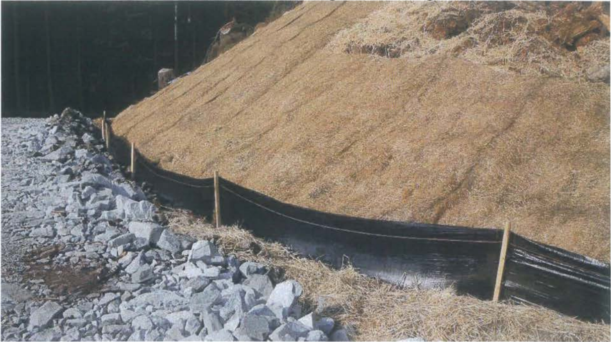
Erosion Control Matting & Silt Fencing
