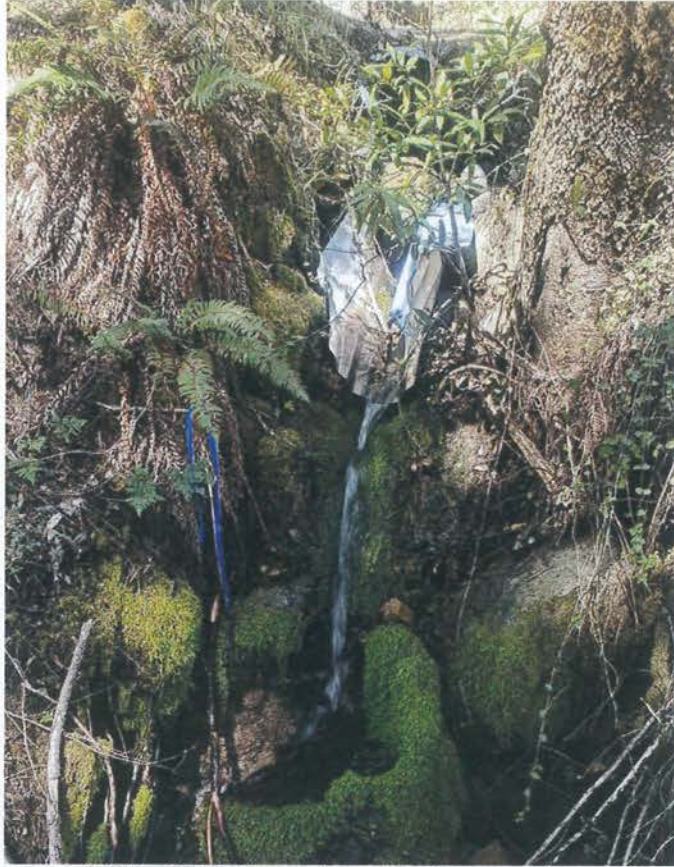
Site 47. Looking at the outlet of the crossing.
