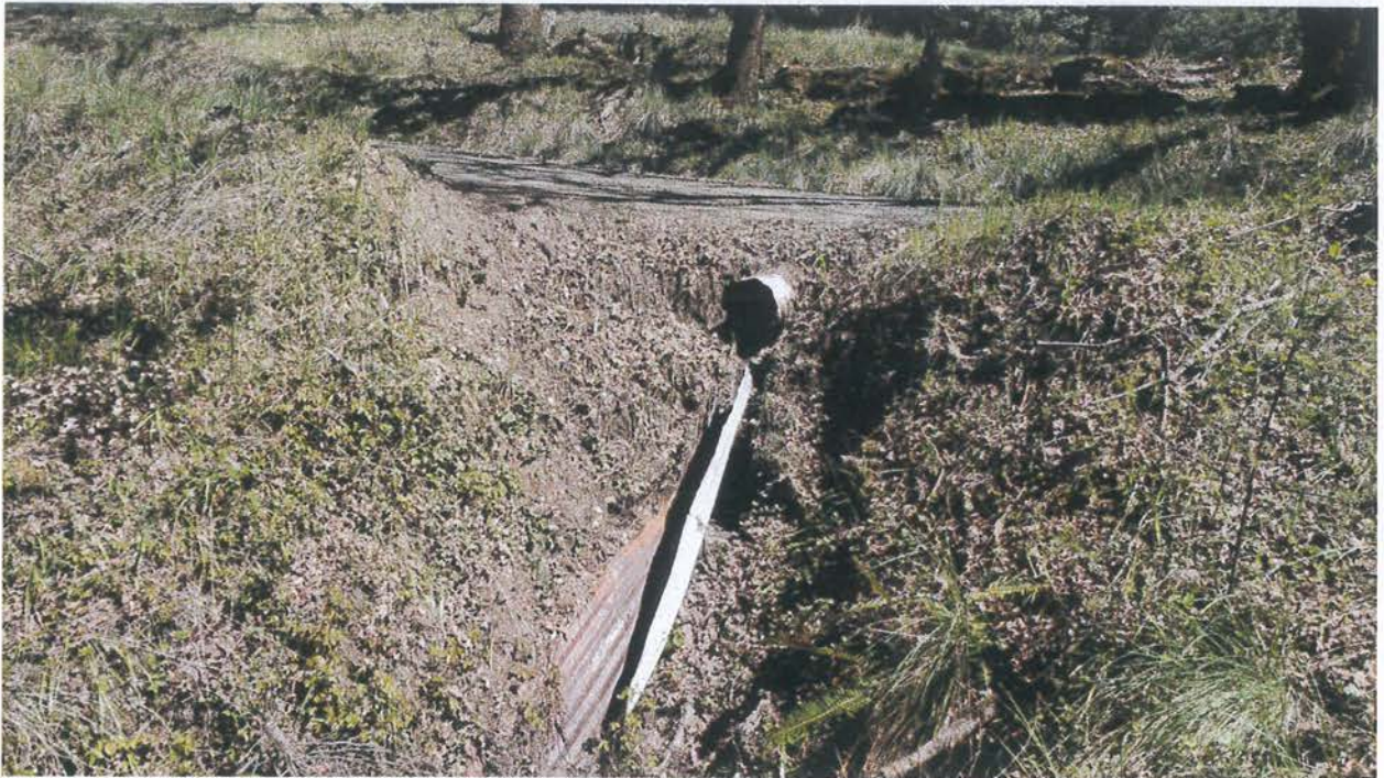
Site 46. Outlet of the ditch relief culvert.
