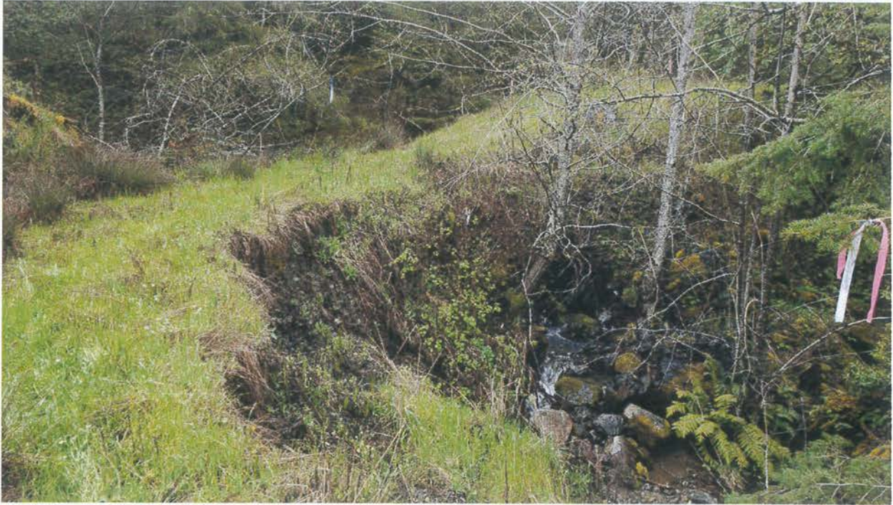
Site 30. Looking at the outlet.
