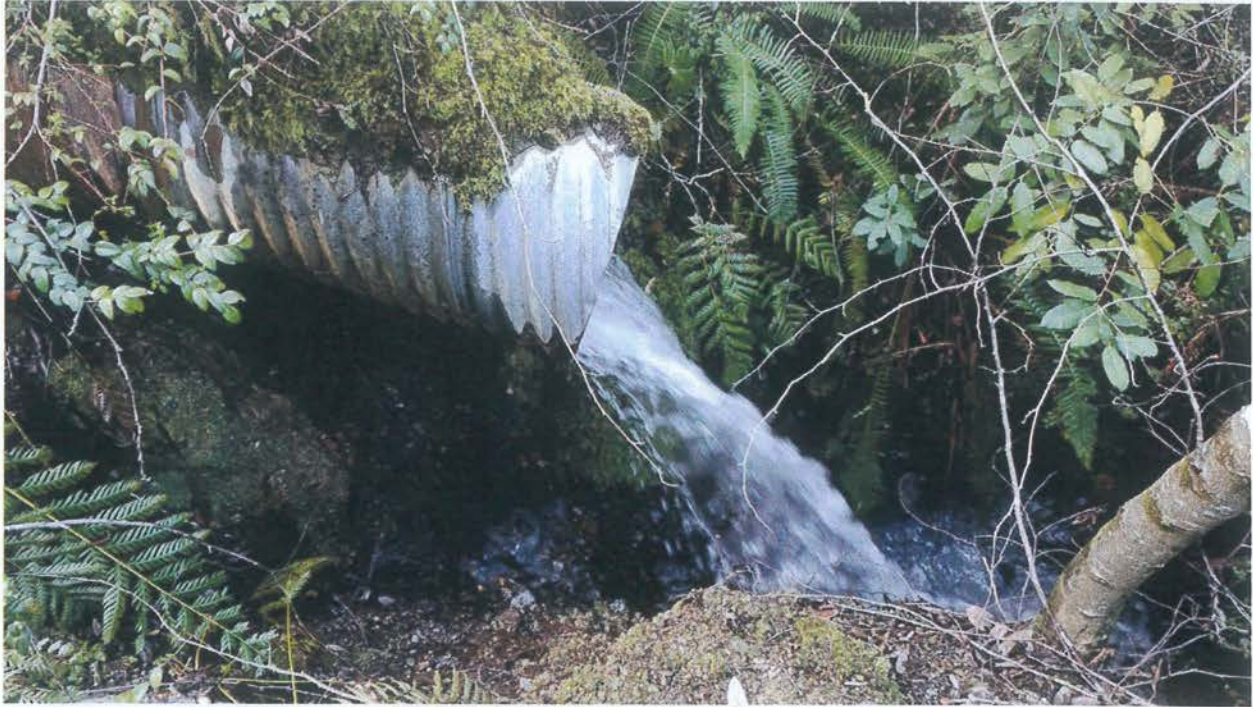
Site 80. Looking at the outlet of the crossing.
