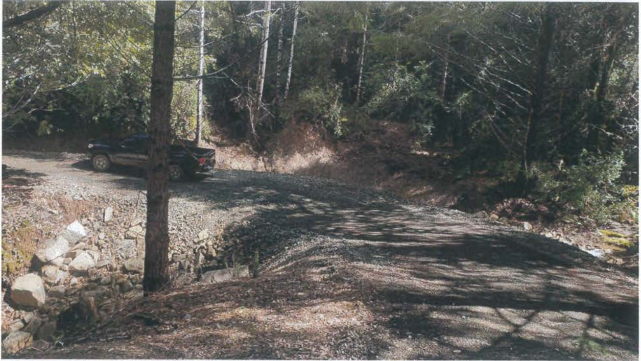
Site 70. Looking south across the newly installed crossing.
