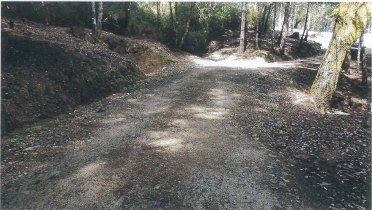
Site 50. Looking north at Site 50. The diverted watercourse from Site 51 is draining down the inside ditch to the left.
