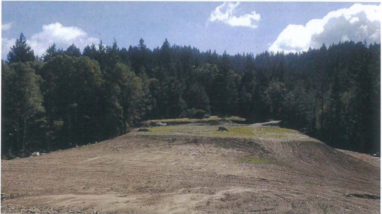
3-acre Conversion Area. Looking west at the conversion area.
