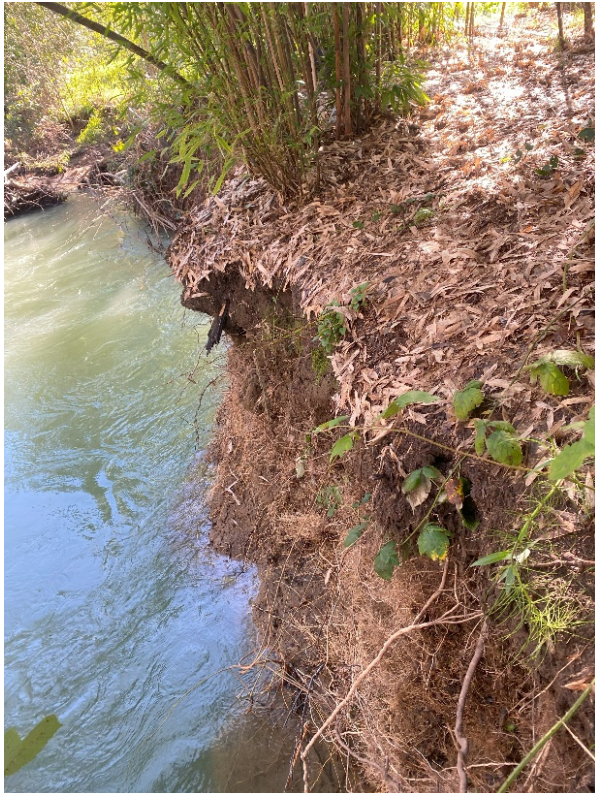
Figure 6: Bank Failure
