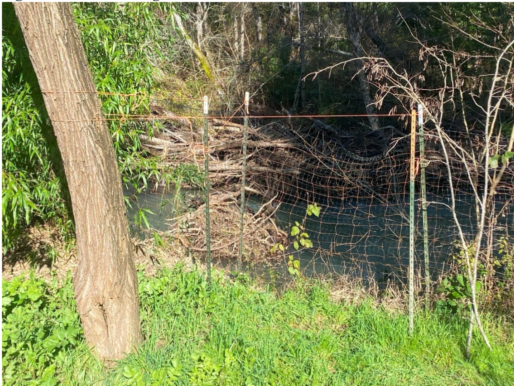
Figure 7: Fence on Edge of Bank Failure
