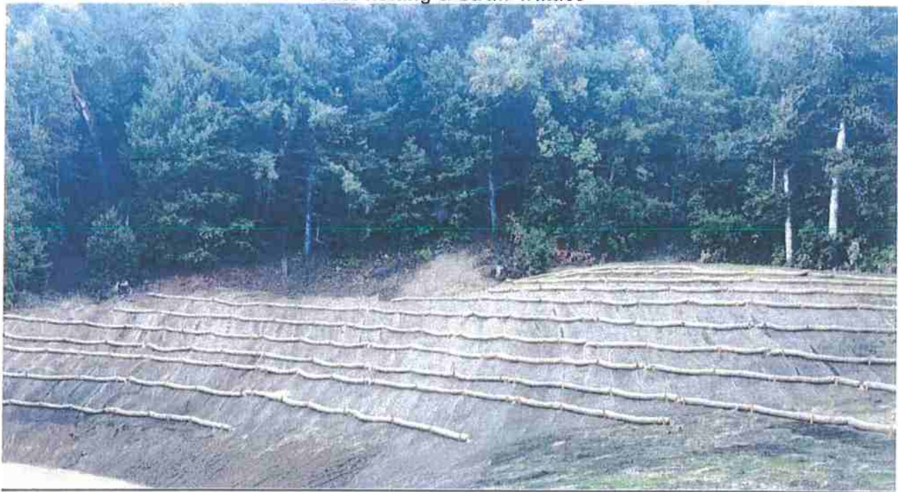
Jute netting & Straw-wattles
