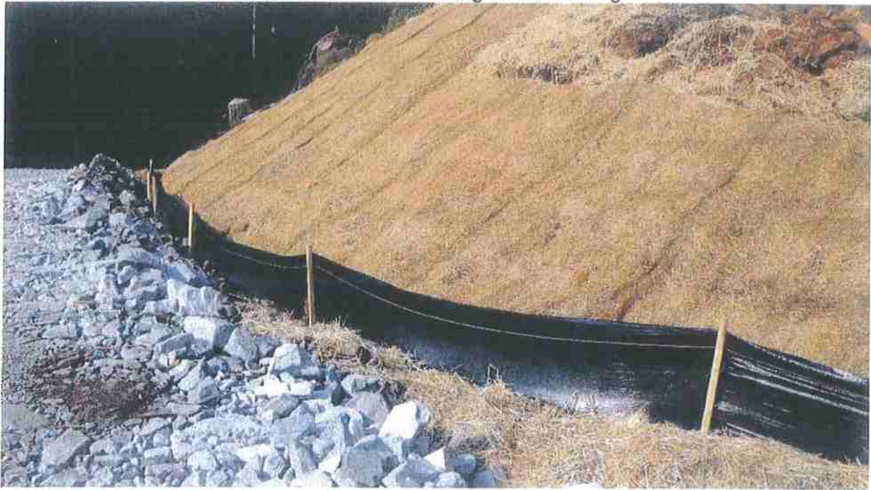
Erosion Control Matting & Silt Fencing
