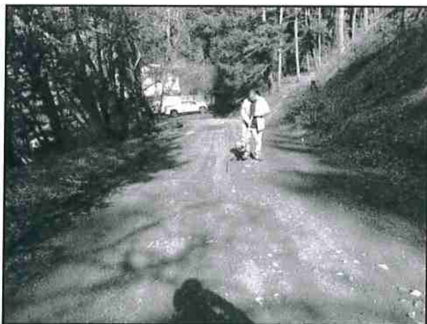
Photo #35 Cobb Rd @ Pullout Looking SW @ Curve
