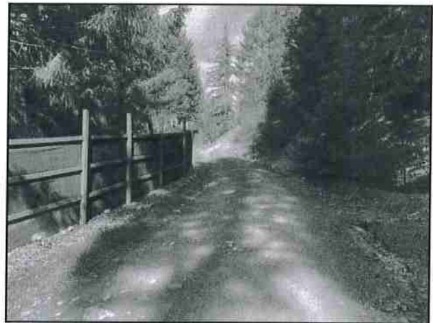
Photo #14 Cobb Rd Looking NW
