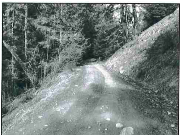
Photo #12 Cobb Rd @ Pullout Looking NW
