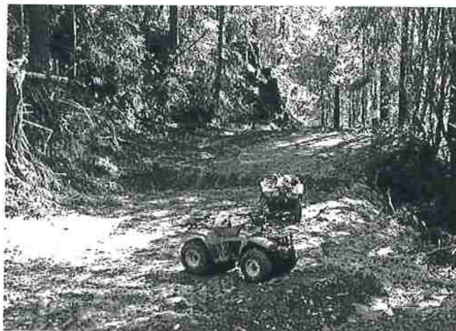
Figure 9. Water bars installed on a road after timber harvesting. Source: Angela Wilson, Central Valley Regional Water Quality Control Board.
