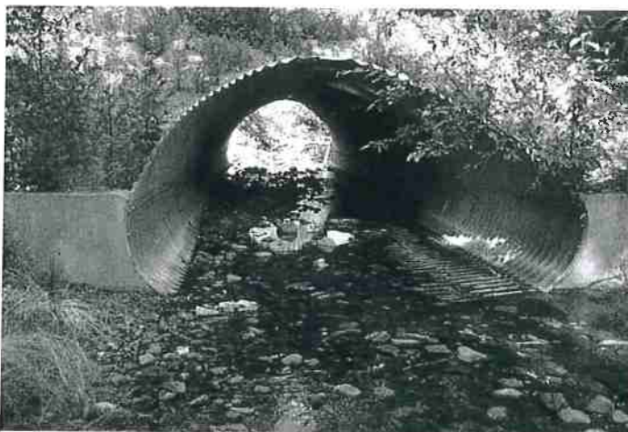
Figure 28. An arched pipe installed on a fish-bearing stream to minimize impacts on fish habitat and migration. Source: Keller and Sherar 2003.
