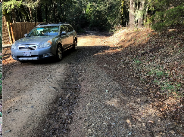
Picture #32 Cobb Rd looking W towards curve.
