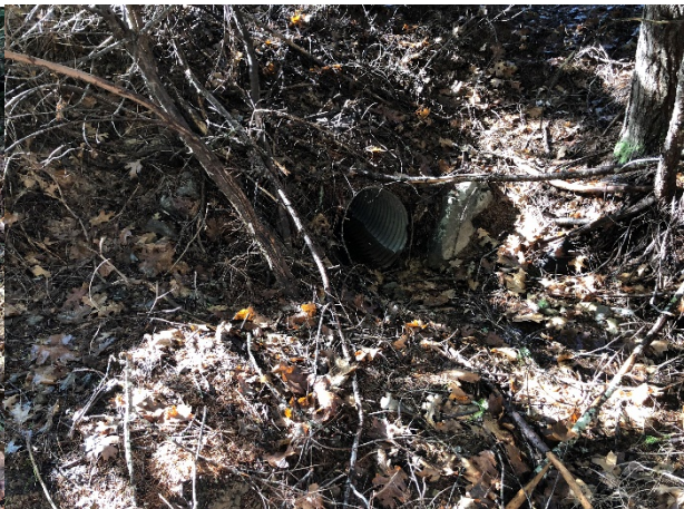
Picture #42 Cobb Rd looking @ inlet of 12" culvert
