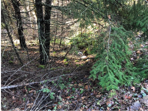
Picture #31 Cobb Rd 12" culvert outlet
