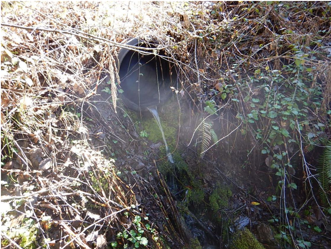
Picture 6. Culvert outlet that needs rocking (3/2/2017)
