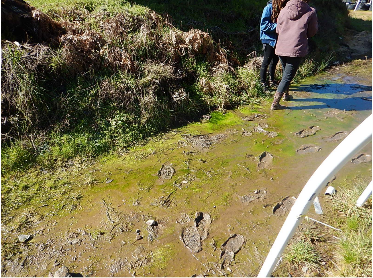
Picture 9. Seeping cut bank and poor flat drainage (3/2/2017)
