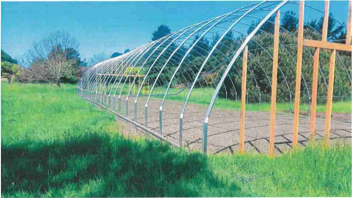
Photo 17. Second hoophouse under construction
