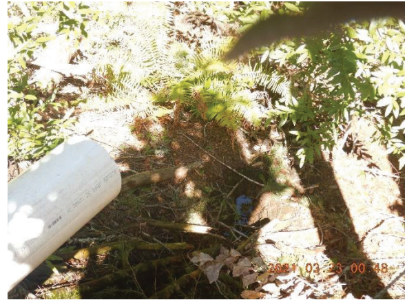
Figure 13. GPS location 449. Trench in previous figure outlets to a pipe that discharges over slope above pond; trench and pipe have potential to carry pollutants to the pond, which provides aquatic habitat and discharges to surface waters.
