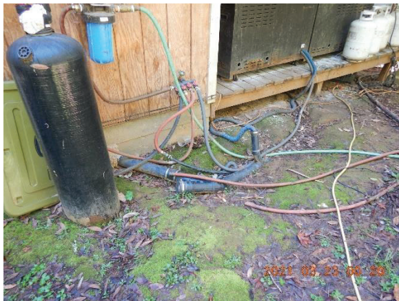
Figure 4. Primary residential facility with waste lines, located within approximately 50 feet of Class II watercourse.
