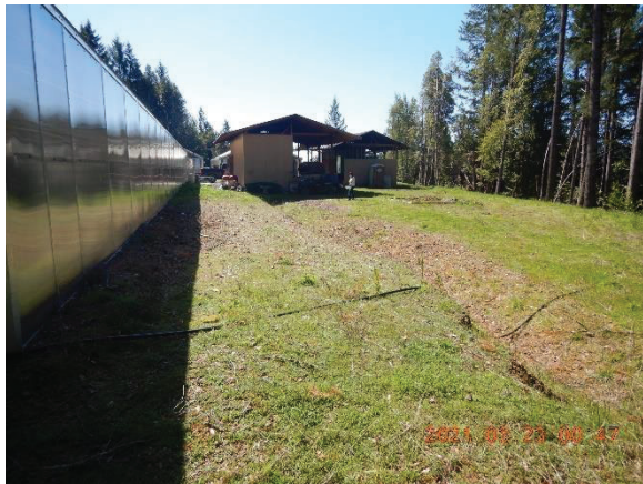
Figure 12. GPS location 448. Gutters catch approx. 12,000 sq ft of greenhouse roof runoff and route it to a trench, located on back side of fuel storage and generator area shown in previous figure. Runoff from the generator area could transport to the trench.
