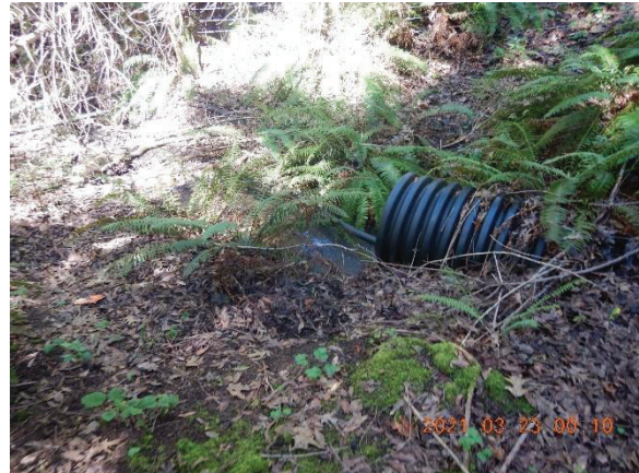
Figure 5. GPS point 445, inlet of 24" which is misaligned located on a Class II watercourse, on a road behind residence, road does not appear to be in use. The culvert was not disclosed in LSA.
