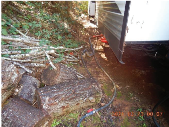
Figure 3. Trailer with waste line presumably to onsite septic system.
