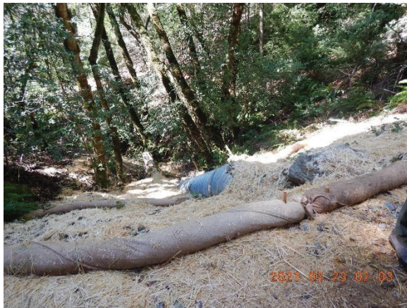
Figure 24. GPS location 462. Crossing 1. Downspout was included in the LSAA but was added during installation of the 36" culvert.
