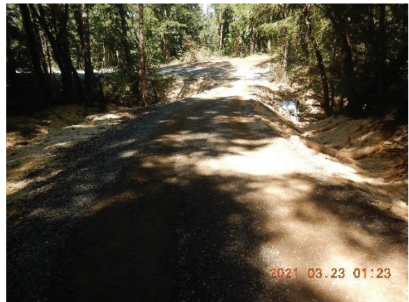
Figure 22. GPS location 455. Looking downslope along road approach to Crossing 3.
