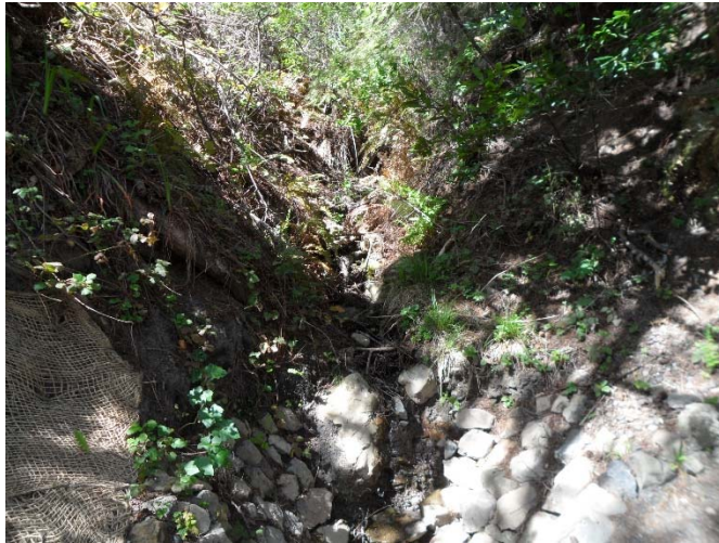
Figure 9. Upslope from Culvert 3/30/2015
