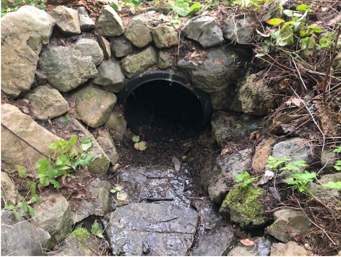
Figure 12. Culvert Post Maintenance 4/17/2020
