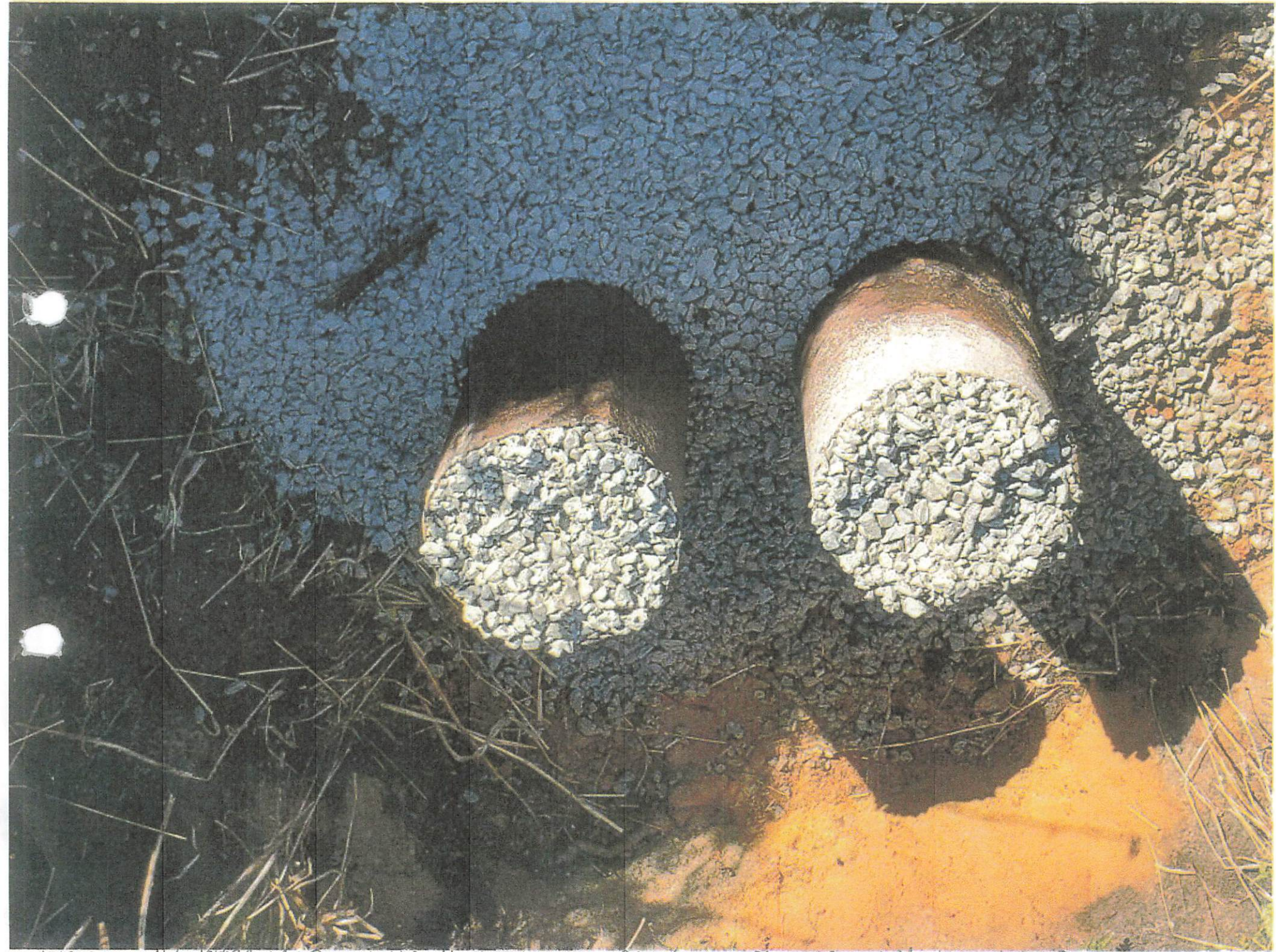
41191a1- Onsite w/ Rich Well Drilling for well destruction. A.M. AP# 308-231-02
