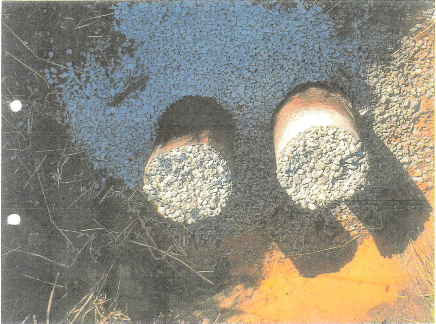
4/14/01 - Onsite w/ Rich Well Drilling for well destruction. AP#308-231-003
