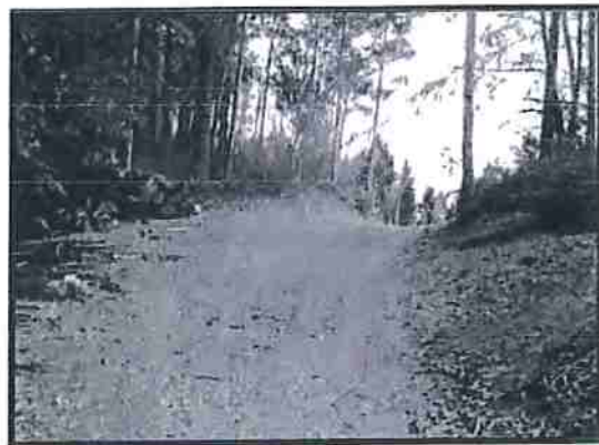
Placement of rolling dip to convey water off of road surface
