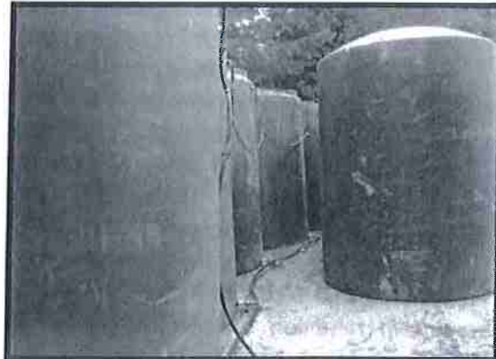
Eight (8) 5000 gallon storage tanks= 40,000 gallon storage
