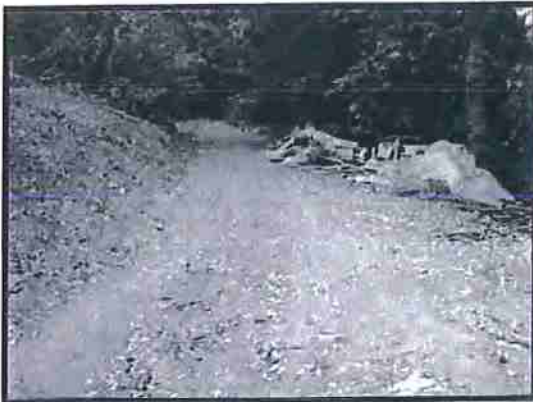
Placement of rolling dip to convey water off of road surface
