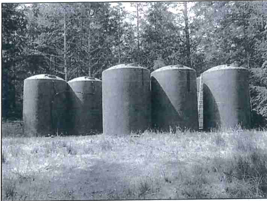
Photo 11 – View of eight water tanks (40,000 gallons total) near the cultivation area on the property.
