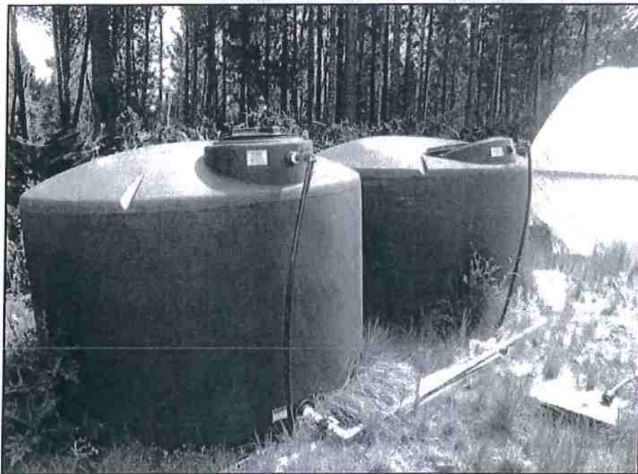
Photo 10 – View of two water tanks (3,100 gallons total) within the cultivation area on the property.
