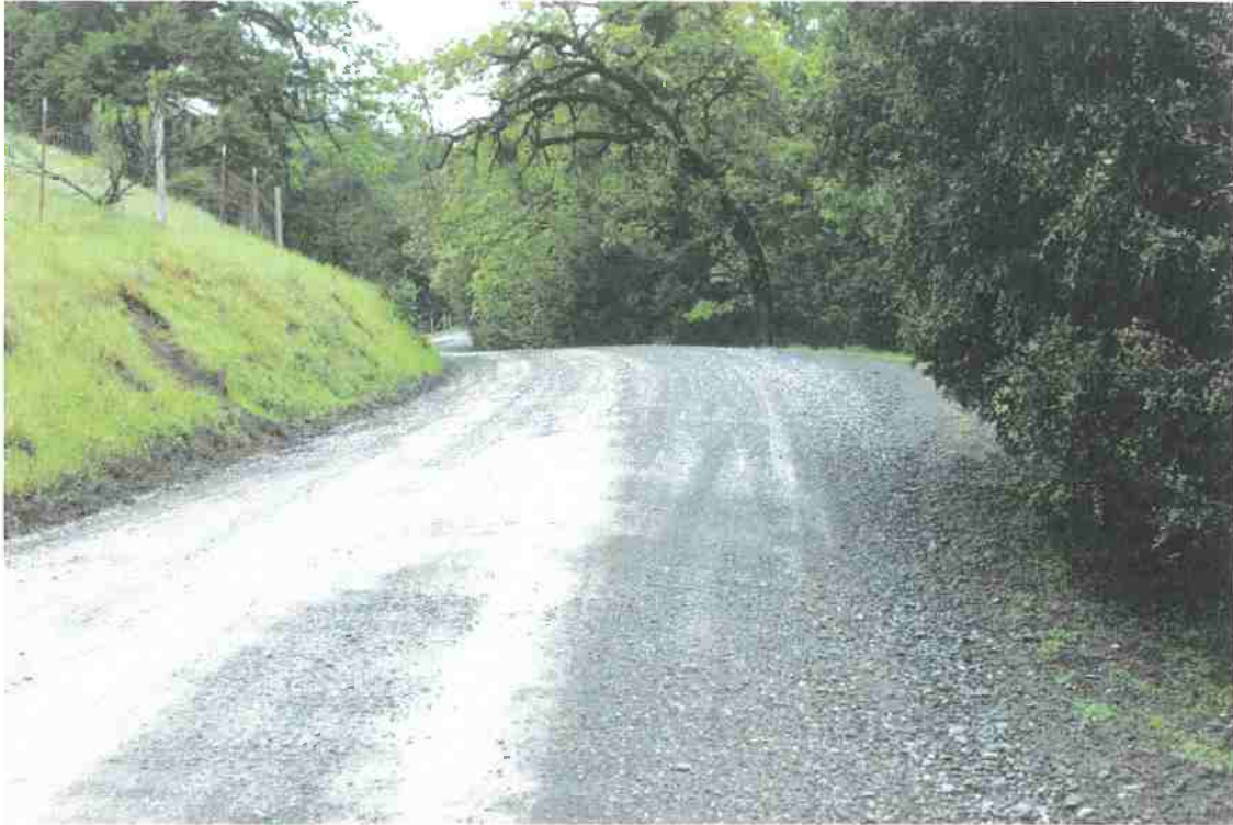
Photo 5. Mile 1.3: Typical lower gradient gravel road segment.
