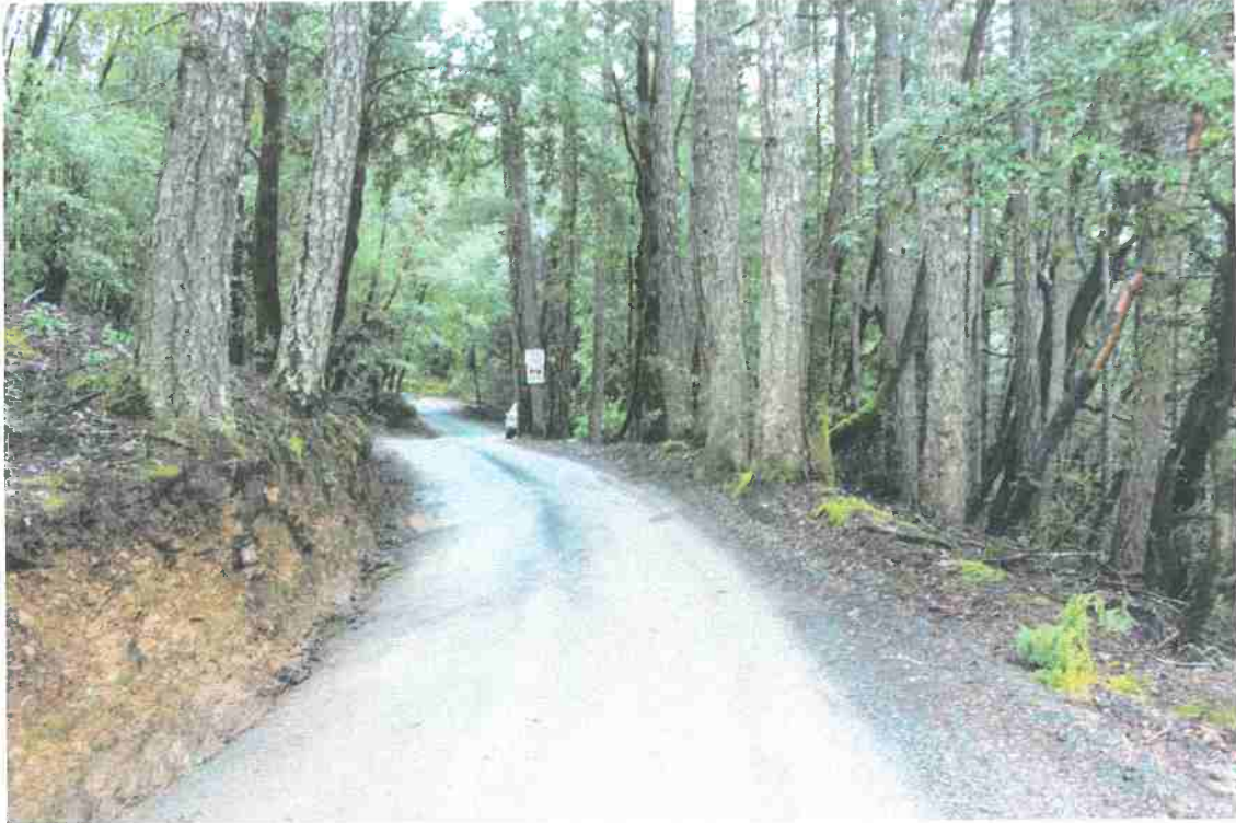
Photo 1. Mile 5.2: 12-ft-wide pinch point with no shoulder at start of private community-maintained road.
