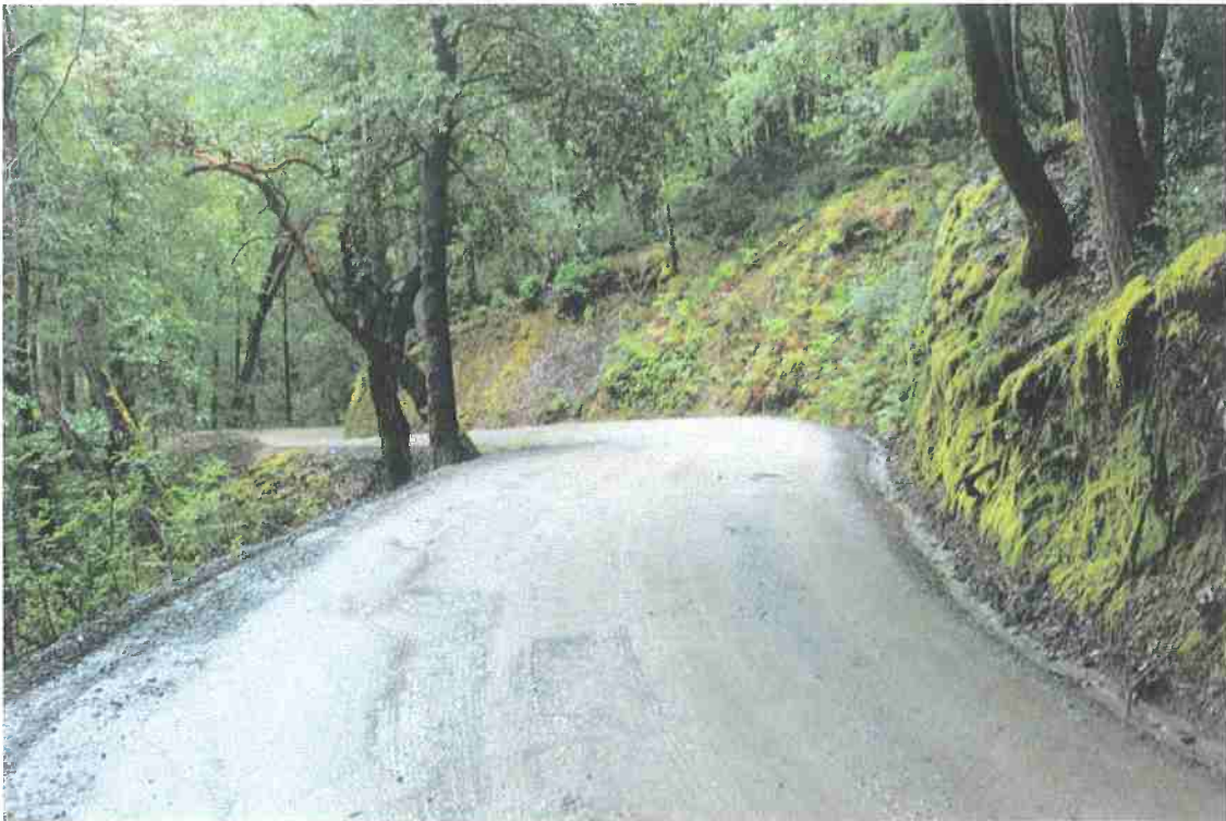
Photo 9. Mile 2.6: Typical 15-ft-wide road segment with good visibility, blind corner in background.
