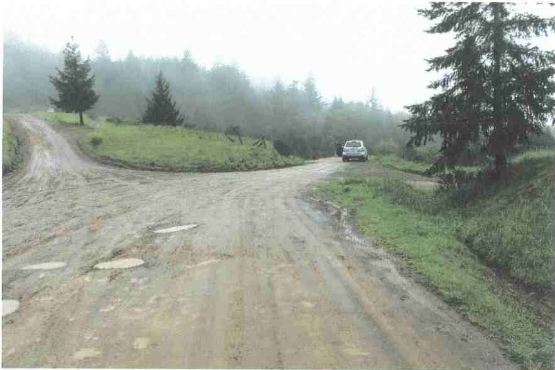
Photo 8. Mile 5.8: 28-ft road width with 2-ft shoulder (end of segment).
