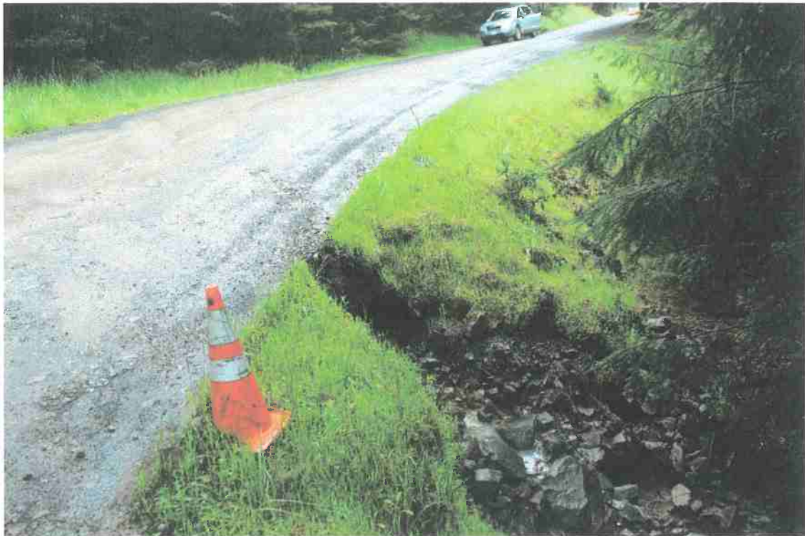
Photo 6. Mile 5.6: Add rock to culvert outlet to prevent erosion of road surface.
