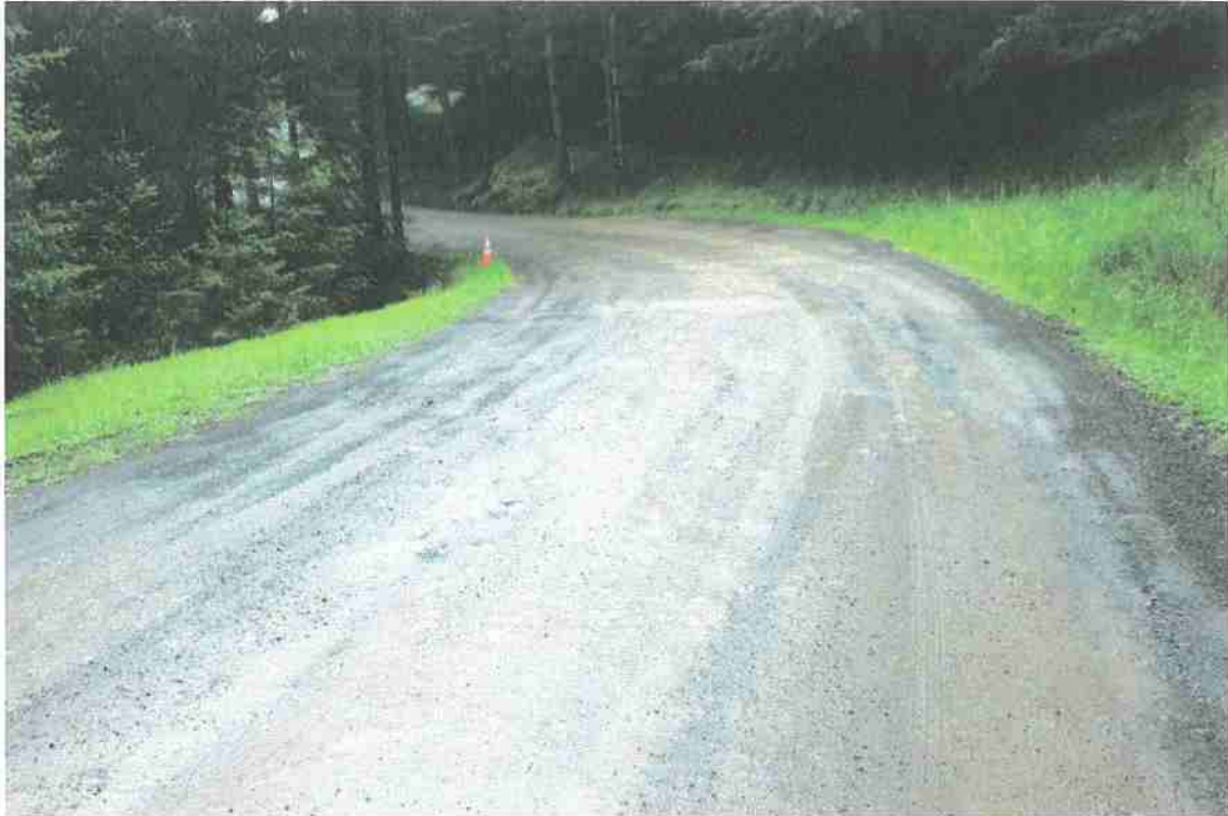
Photo 5. Mile 5.6: 20-ft road width with 2-ft shoulder.
