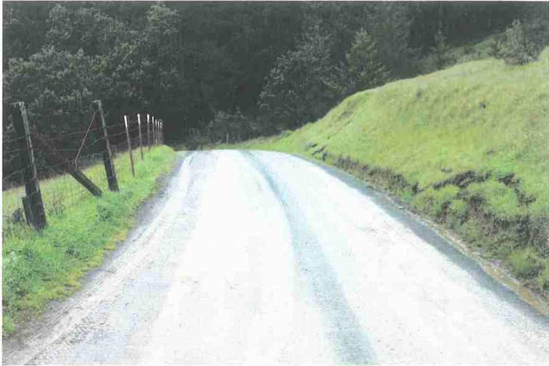
Photo 3. Mile 5.4: 12-ft-wide pinch point with no shoulders.
