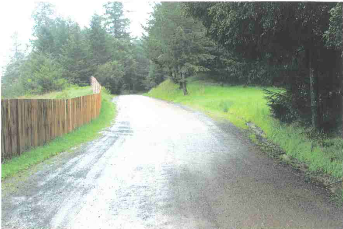
Photo 4. Mile 5.5: 20-ft road width with 2-ft shoulder.
