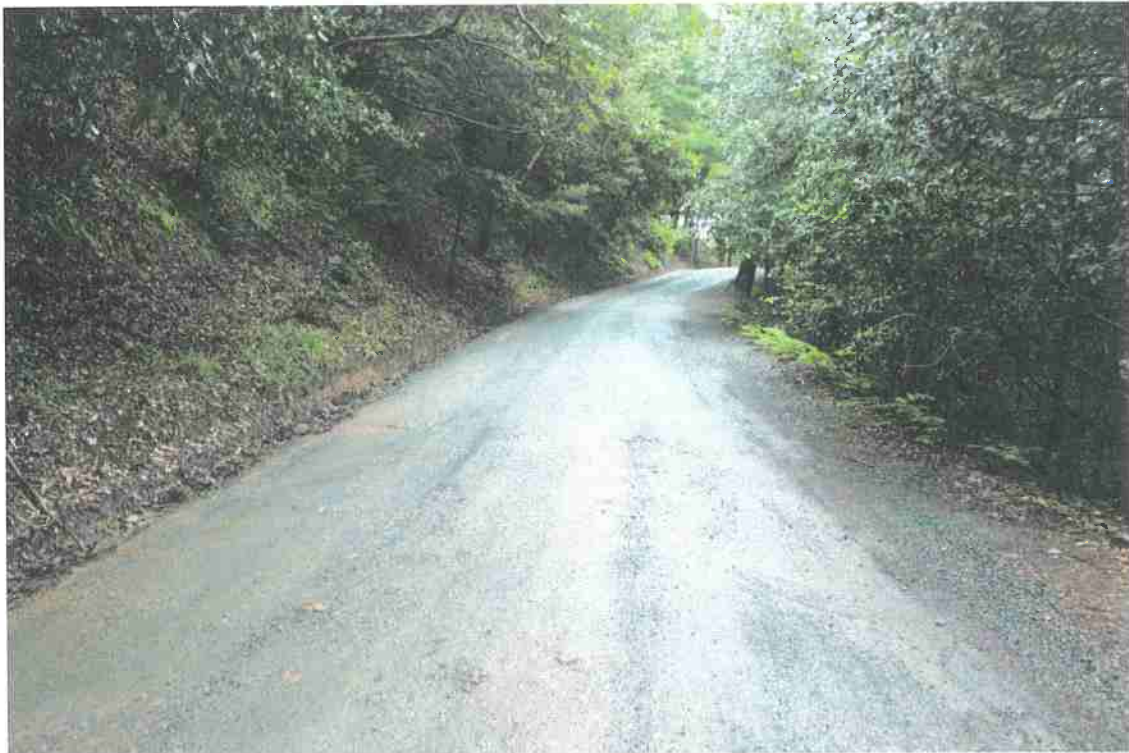
Photo 2. Mile 5.3: 18-ft road width with 2-ft shoulders.
