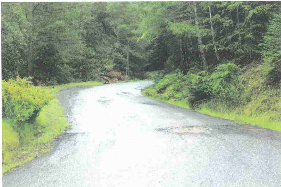
Photo 2. Mile 0.2: Typical steeper gradient paved road segment.
