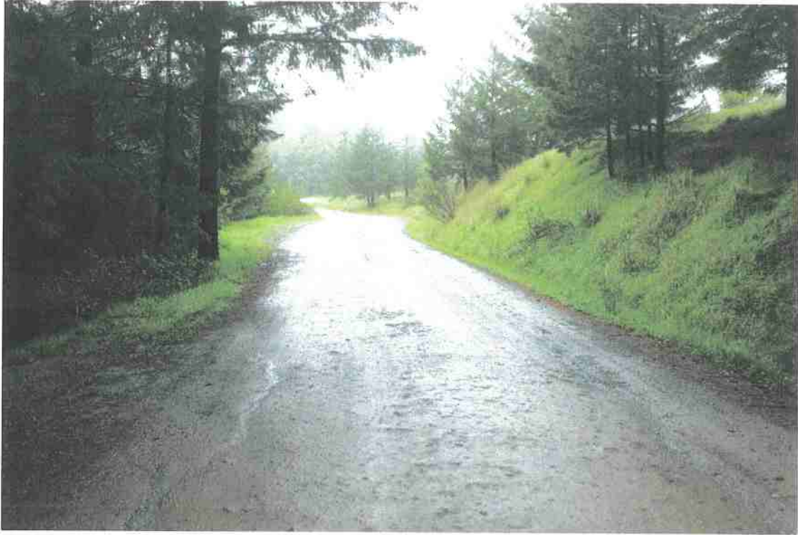
Photo 7. Mile 5.7: 20-ft road width with 2-ft shoulder.
