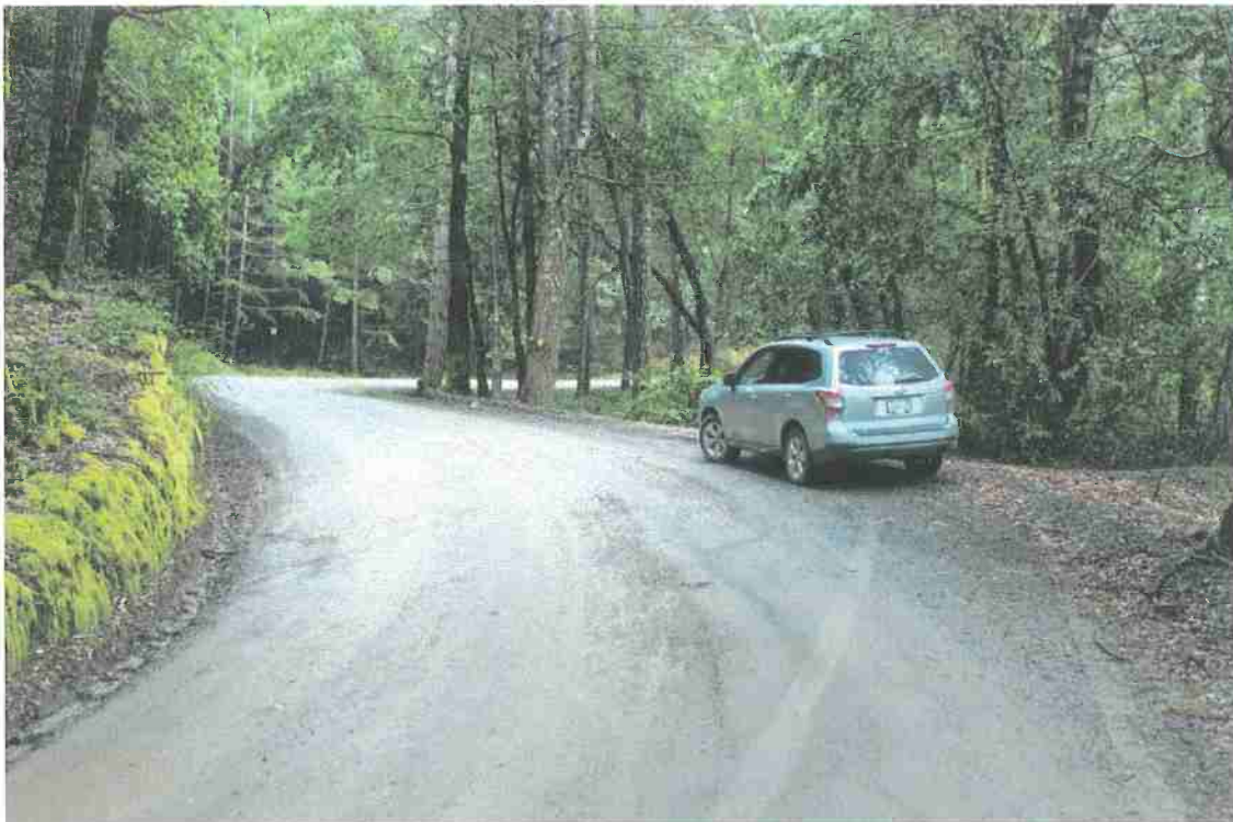
Photo 10. Mile 2.6: Typical 18-ft-wide road segment with turnouts.
