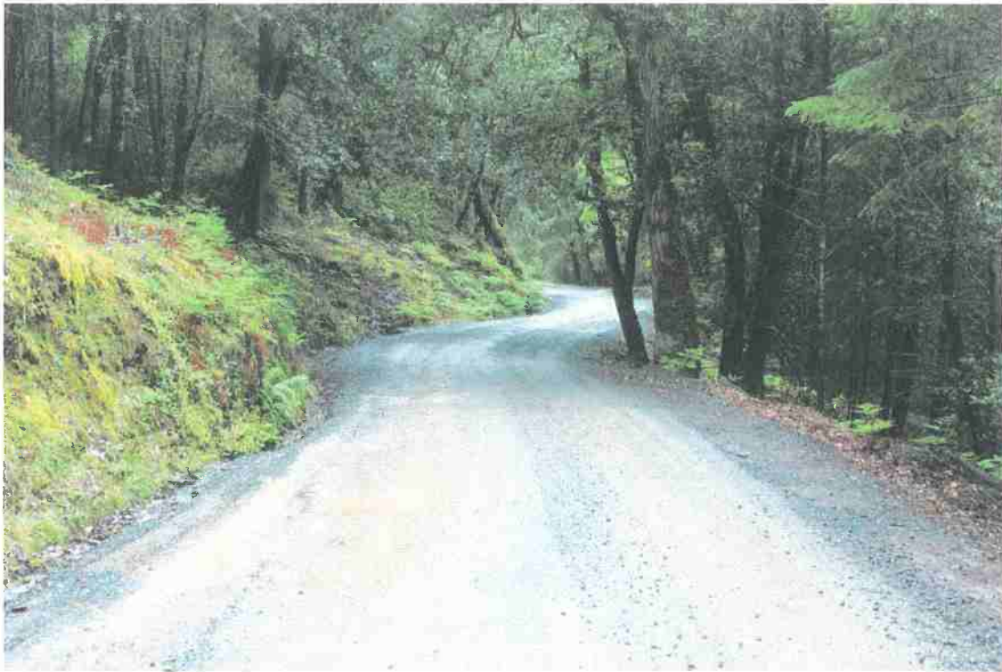
Photo 7. Mile 2.0: Typical steeper segment with Pinch Point 4 in background.
