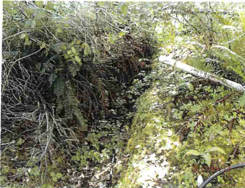
Photo 1- View of POD #1, a dug out trench with a gravity fed \frac{3}{4} inch poly pipe
