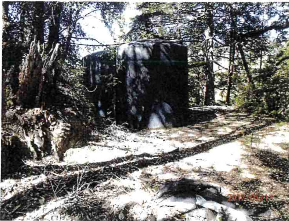
Photo 8- View of the two 3,000 gallon water tanks that are filled from the cistern.
