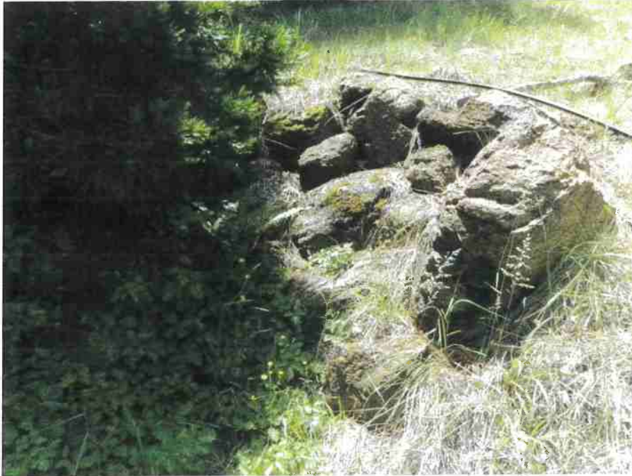
Photo 1- View of POD #1, spring intake on neighboring parcel, a non-jurisdictional water source.
