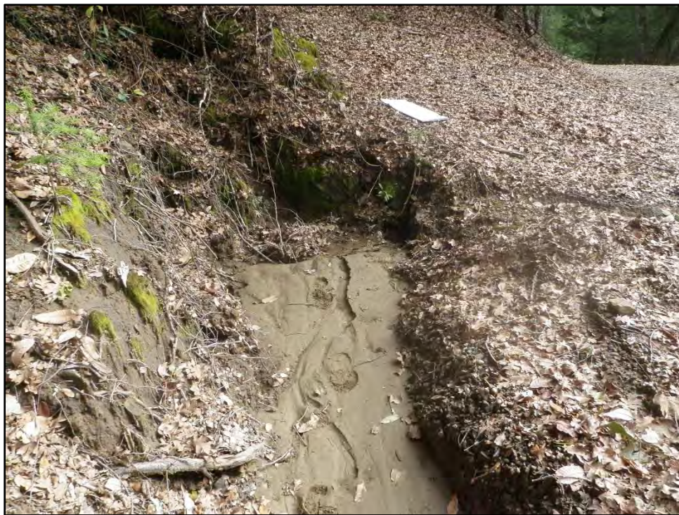
Photo 6 – Project #3, View of the inlet of SC #2 from the right road inboard ditch, which is actively delivering fine sediment to the crossing.
