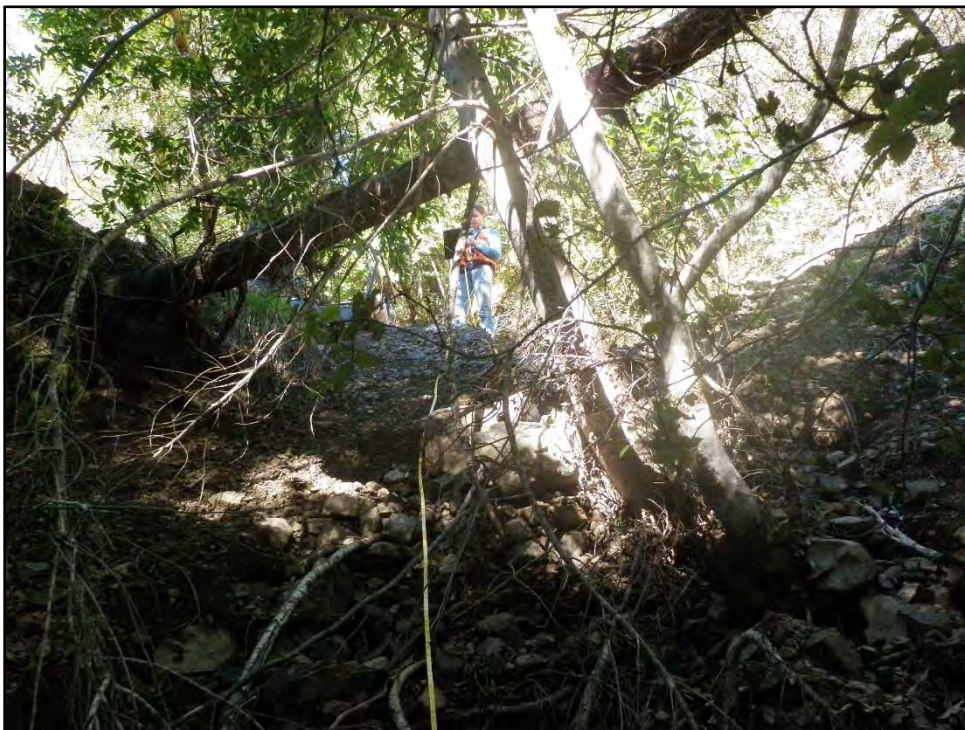
Photo 14 – Project #7, View from the base of fill at SC #7 looking upslope at the outboard fill face.
