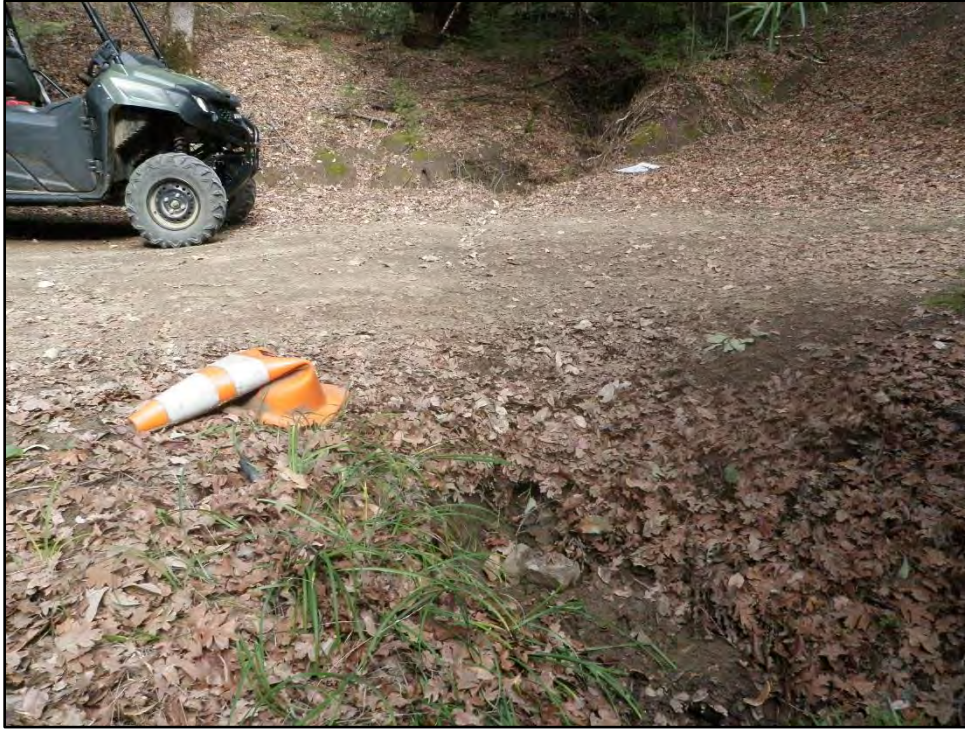
Photo 7 – Project #3, View looking upstream from the outlet of SC #2.
