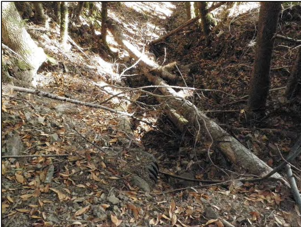
Photo 16 – Project #8, View looking downstream at SC #8 culvert outlet.
