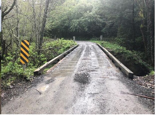
Photo #8 One Lane Bridge @ Chambers Rd & Mill Creek
