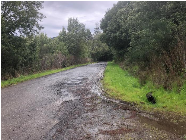
Photo #3 Intersection of Chambers Rd & DW Looking East
