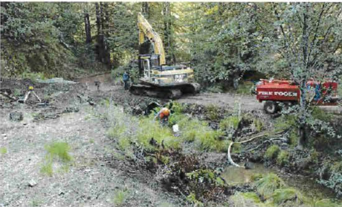
FIGURE 199. For larger streams, pump trucks, large pumps or multiple small pumps can be used to pump streamflow around project work sites. Here, a pump truck is used to temporarily divert flow in a fish bearing stream where dual culverts are being replaced with a riser bridge. Young fish were removed from this fish bearing stream before project work started.
