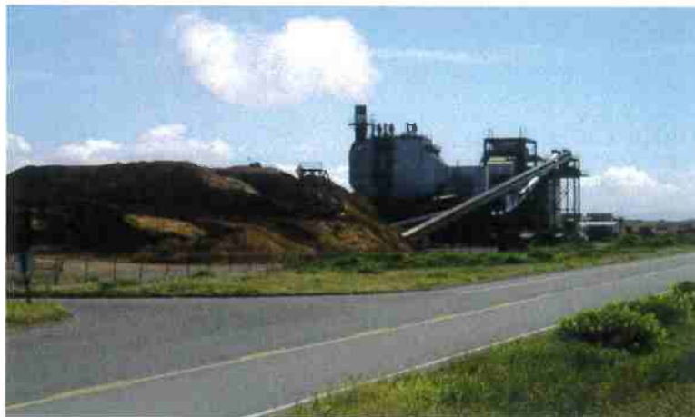
Photo 4: Overview of the project site looking south along New Navy Base Road.
