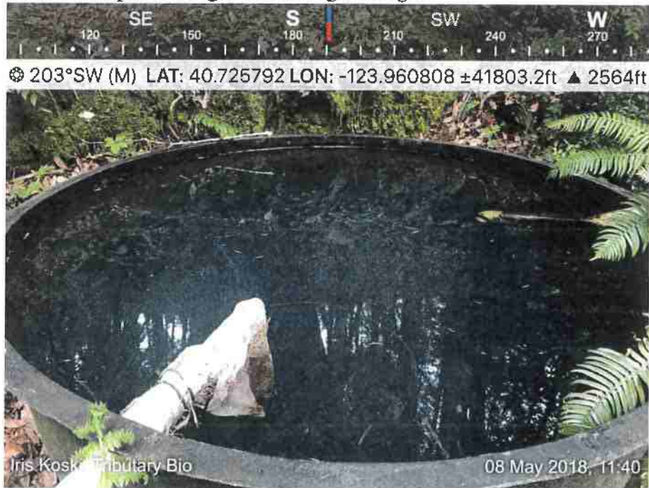
Photo 8. Open 500-gallon storage trough.
