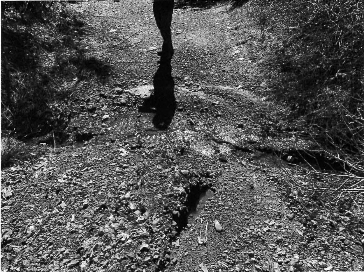
Photo #3: Photograph showing the structureless watercourse crossing identified as Site 15.
