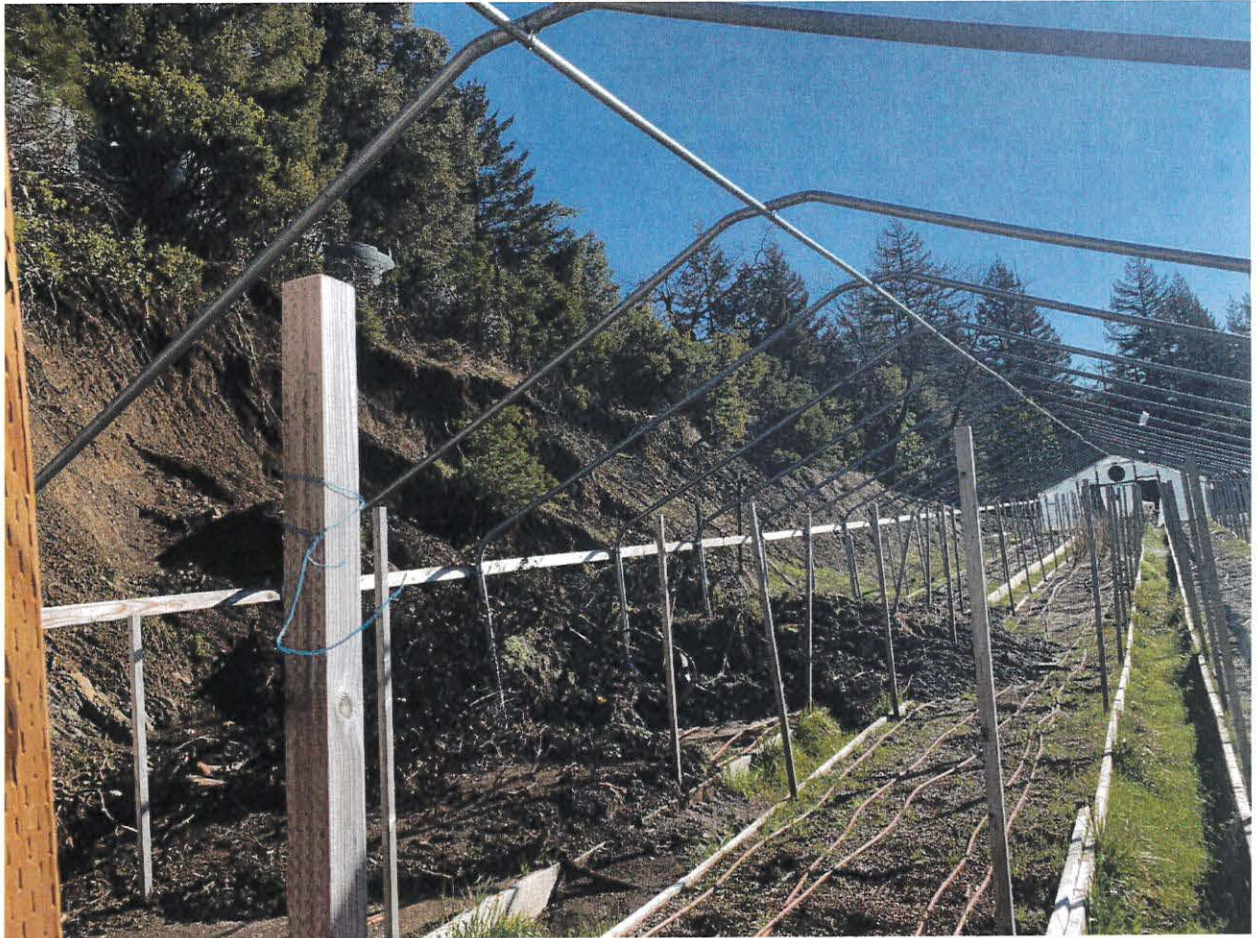
Photo #2: Photograph showing the cut-bank slump identified as Site 22.
