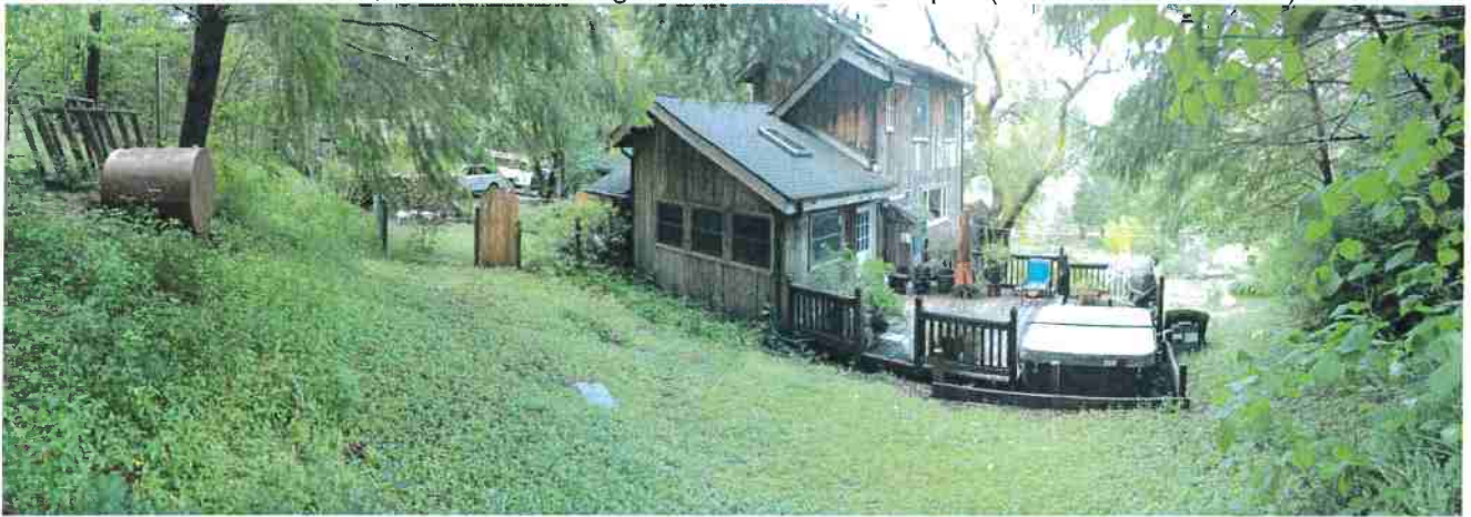
Photo 6. Site B; northeast corner looking southwest.
