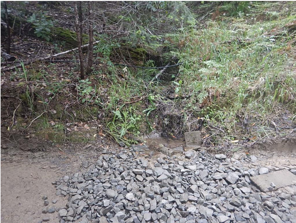
Inboard edge of road at rocky crossing, looking upstream (Project 1)
