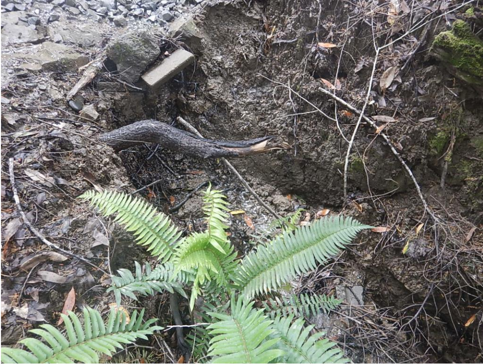
Outboard edge of road at rocky crossing, looking upstream (Project 1)
