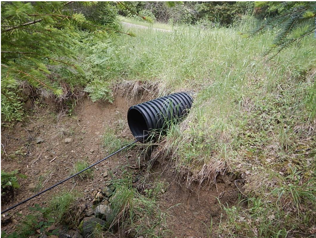
Stream crossing outlet (Project 2)
