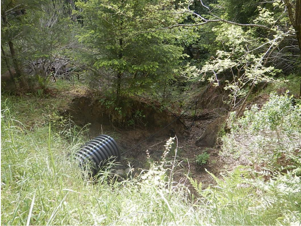
Stream crossing outlet, looking downstream (Project 2).
