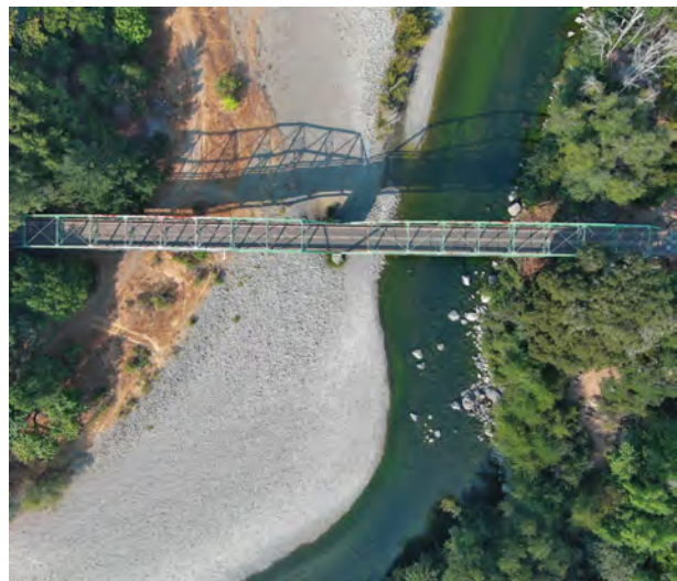
UAV imagery (above) can identify conflicts with existing utilities and infrastructure and provide more thorough pre-construction condition documentation.
