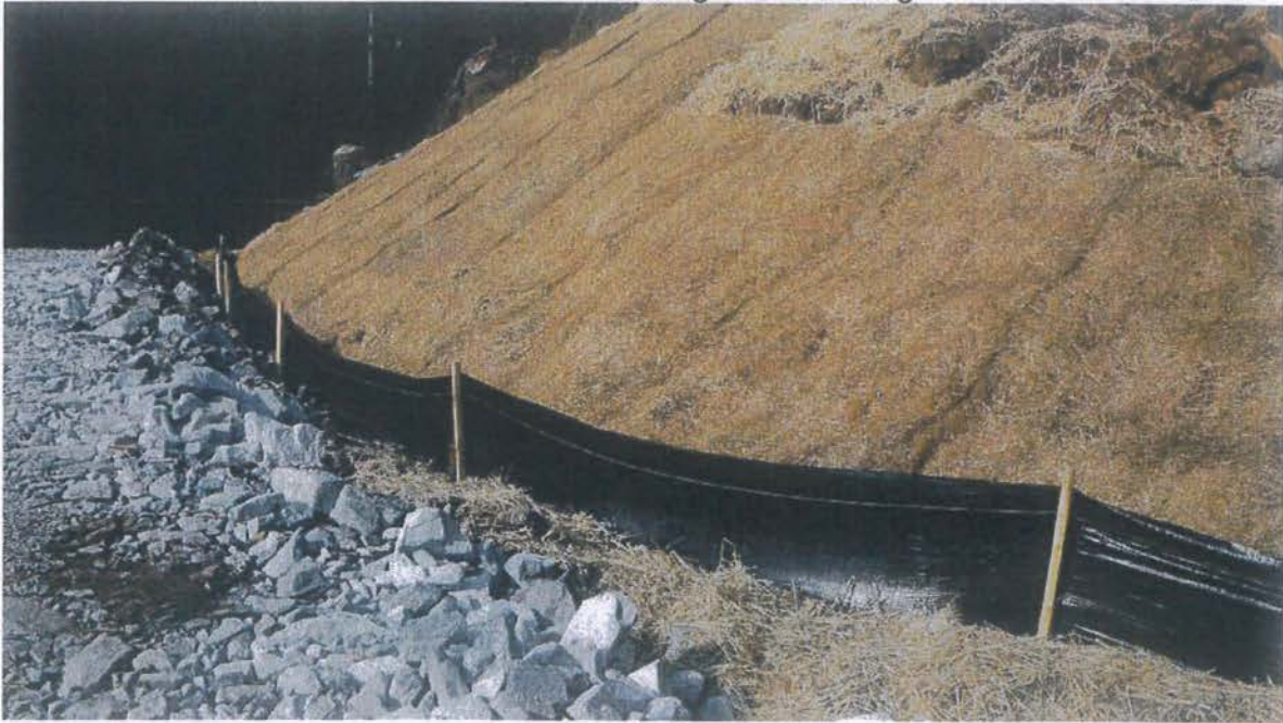
Erosion Control Matting & Silt Fencing
