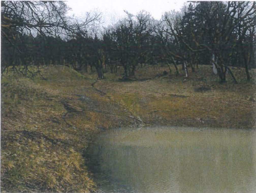
Off-stream pond with a pipe feeding from the surface water diversion above. Riling is presently leading into the pond.
