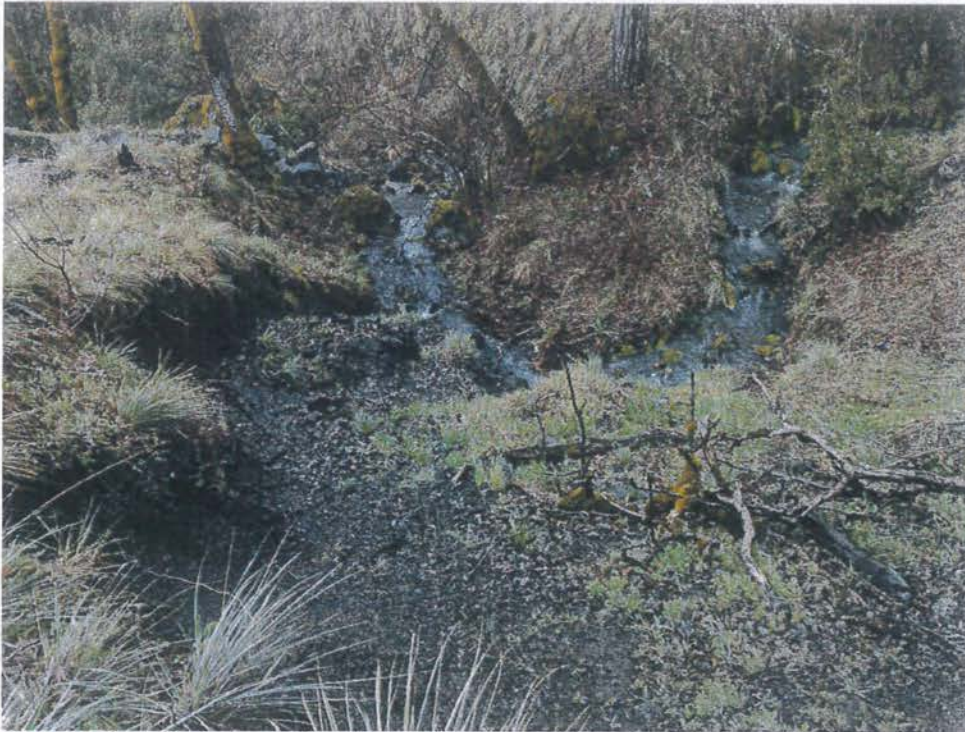
Site 09 of the instream bank slope failure. This site should be examined by a licensed geologist or engineer immediately.
