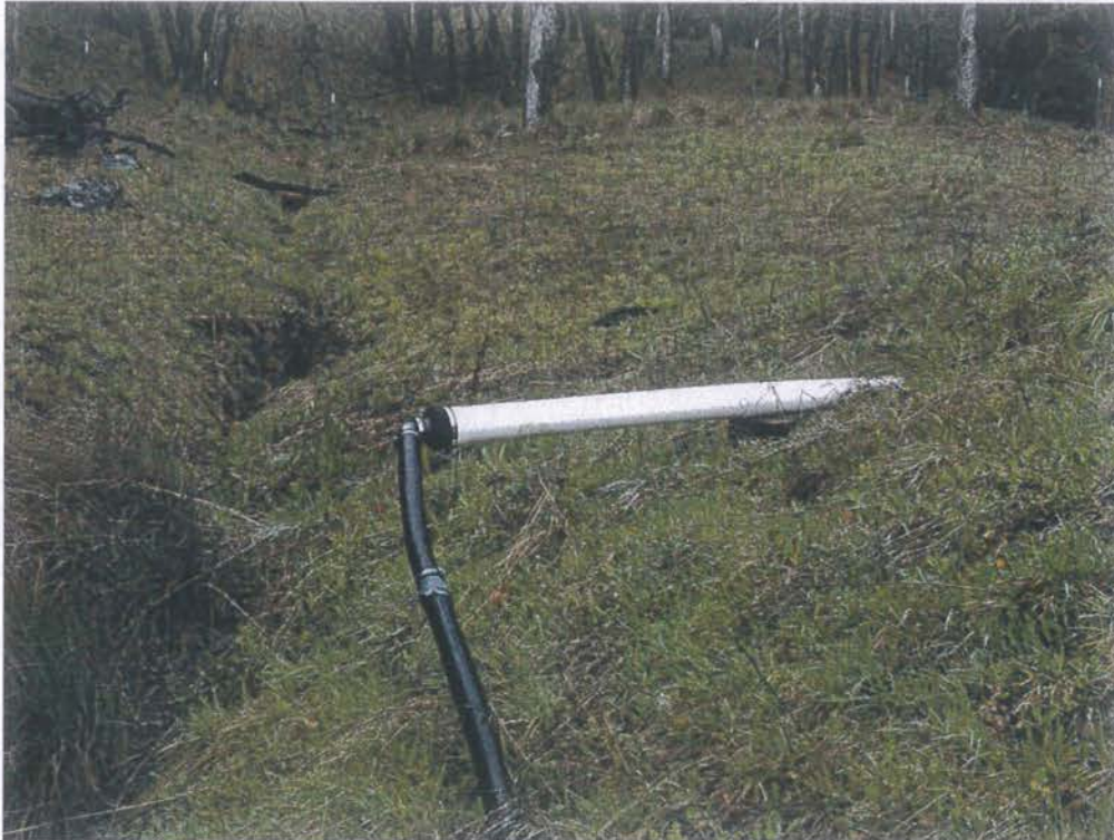
French drain surface water diversion.
