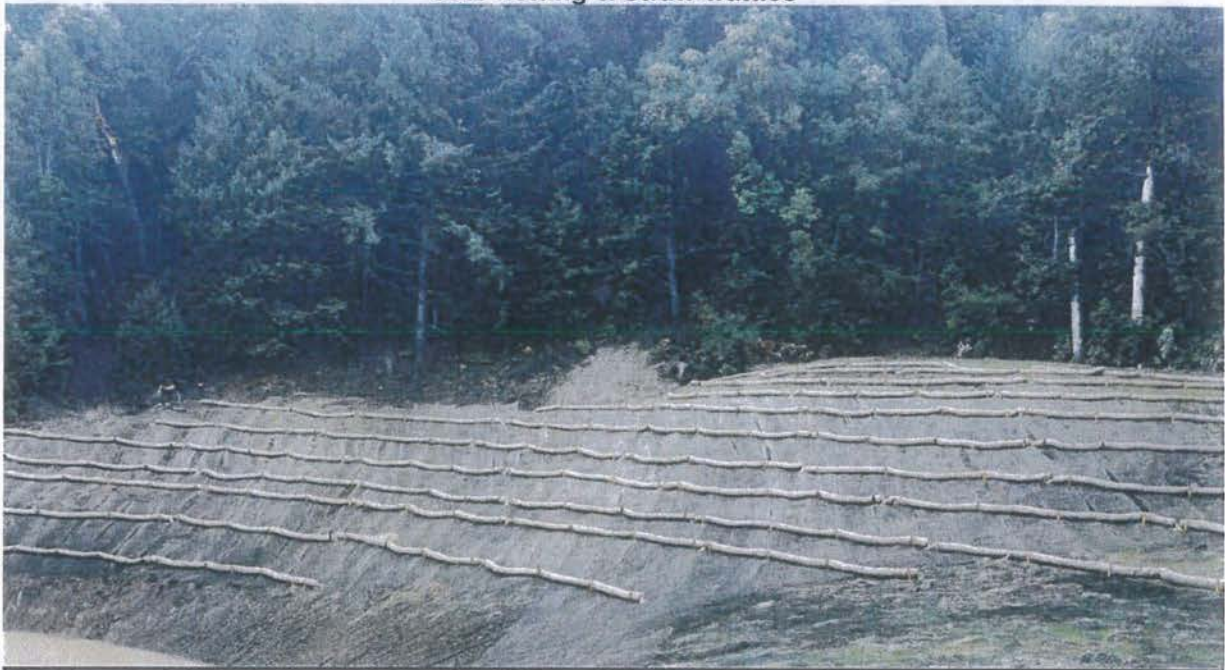
Jute netting & Straw-wattles
