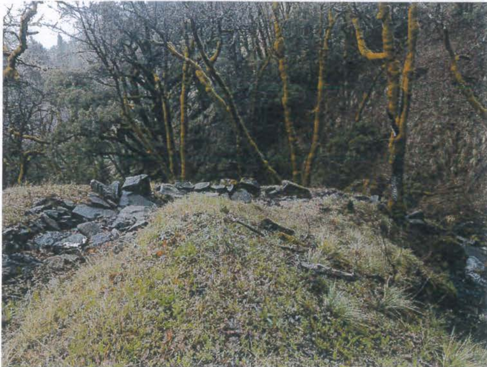
Rocked spillway the drains into a Class II watercourse.
