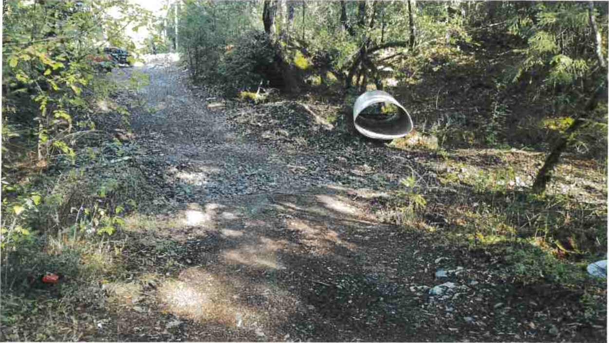
Photo looking north at Site 03.
