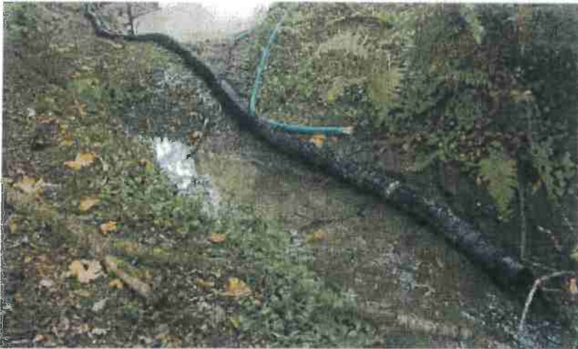
FIGURE 197. Flex pipe stream diversion around a road construction site. The inlet to this 8 inch diameter flex pipe inlet collects clear streamflow from a retention dam above the project site and gravity feeds it around the project area and back into the natural channel downstream from construction work (see photo).
