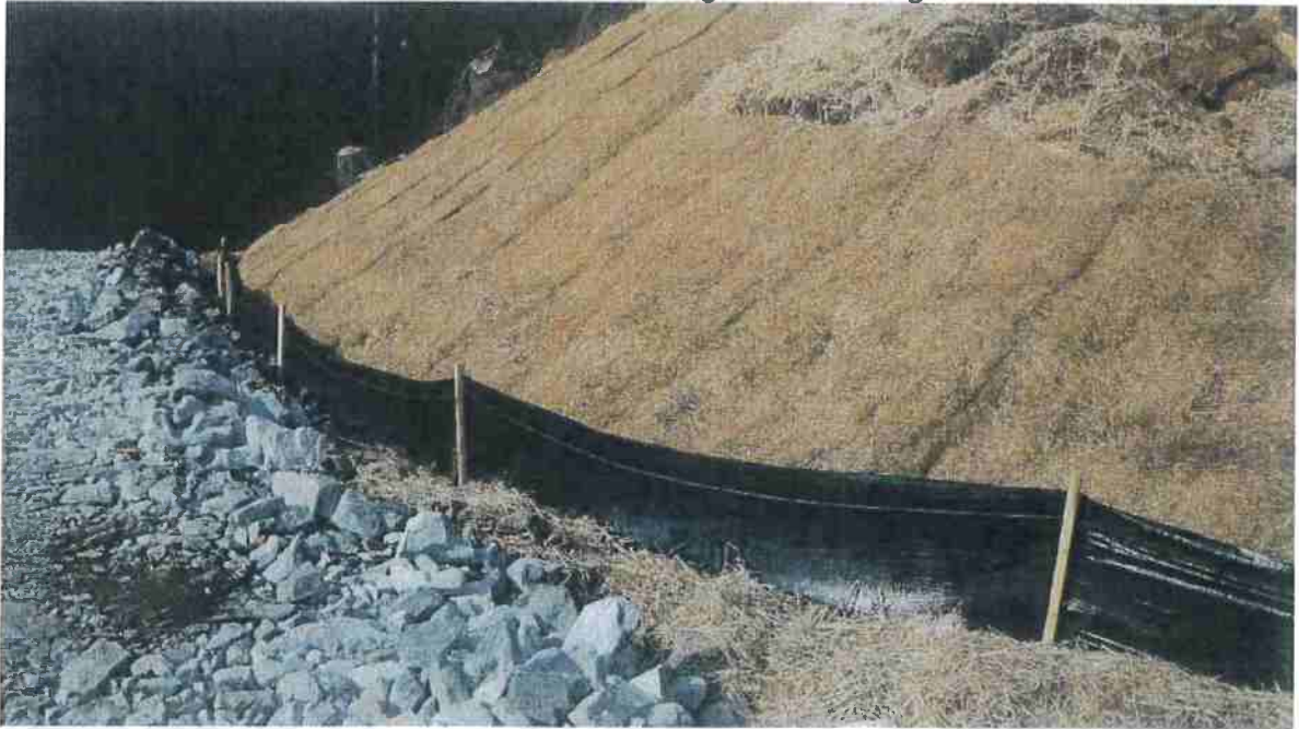
Erosion Control Matting & Silt Fencing
