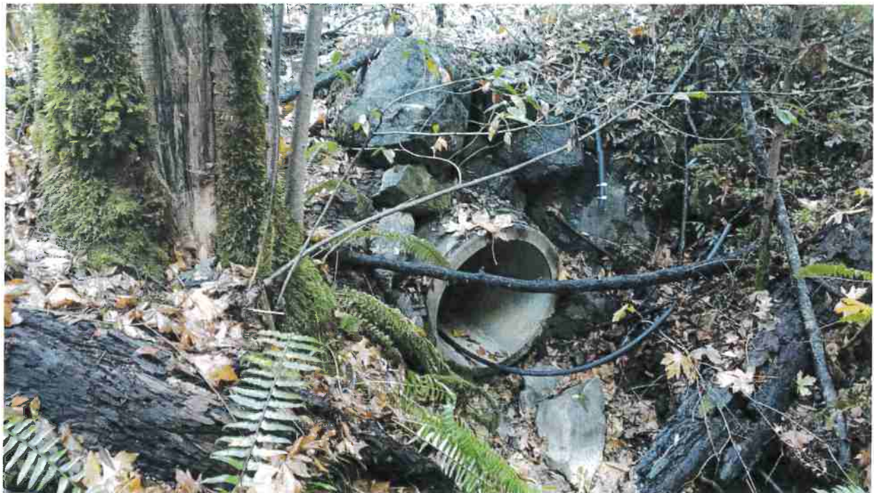
Photo of the outlet of the watercourse crossing at Site 13.
