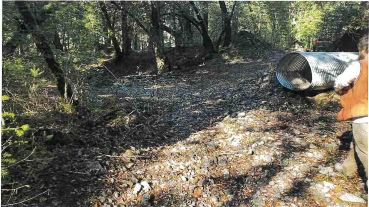
Photo looking down stream at Site 03.
