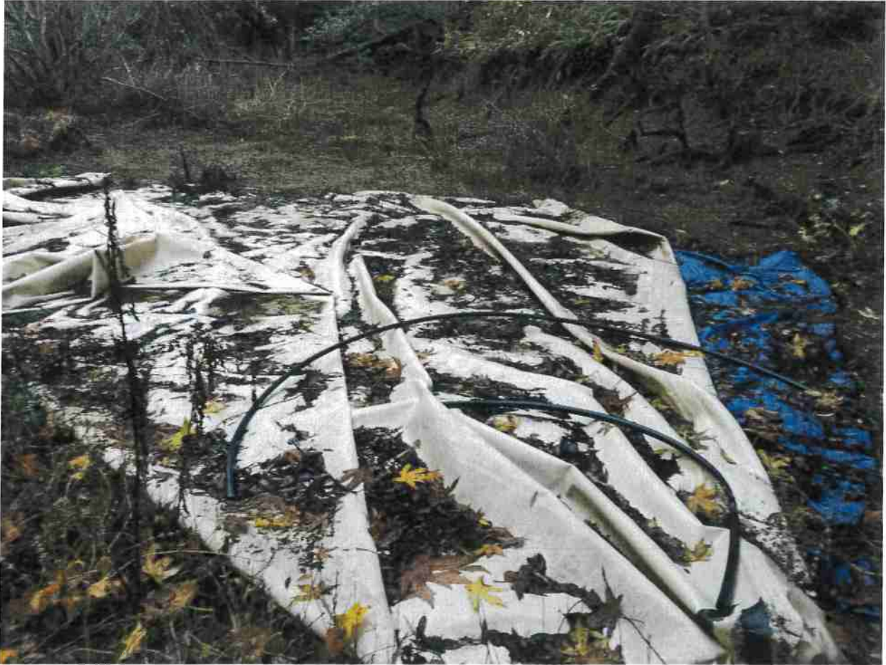
Photo of the water storage bladder at Site 12.
