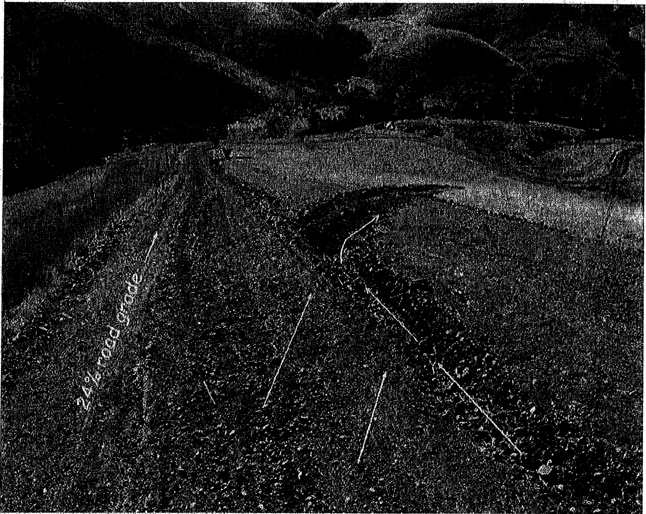
FIGURE 55. Steep roads that go straight up or down a hillside are very difficult to drain. This steep, full line road developed a through out cross section that was drained using lead out ditches to direct runoff off the road and onto the adjacent, vegetated hillside. The road was "outloped" to drain runoff to the right side, and the lead out ditch was built slightly steeper than the road grade, to be self-cleaning. Four lead out ditches have been constructed at 100-foot intervals to the bottom of the hillside.
