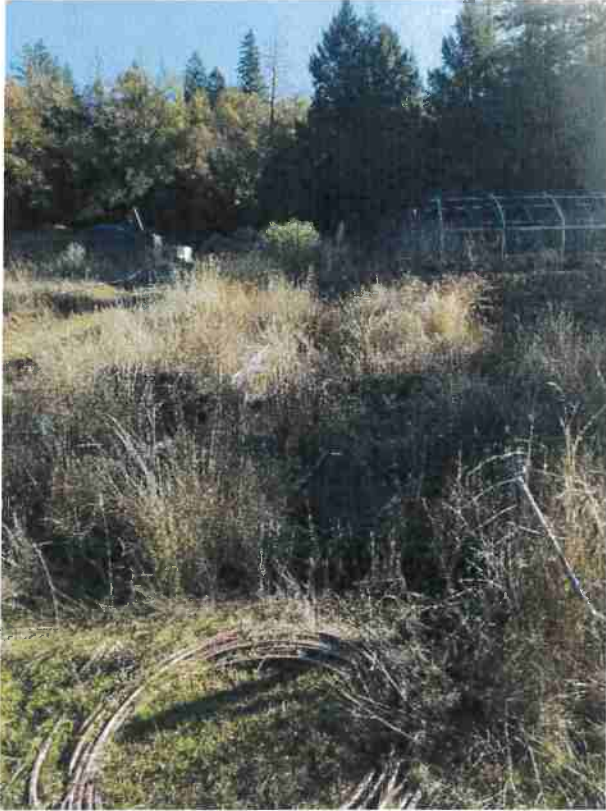
Photo looking up channel from the inlet of the watercourse crossing at Site 17.
