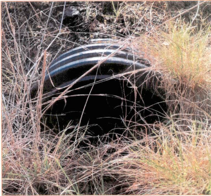
RP9) Clean and maintain DRC inlet.
