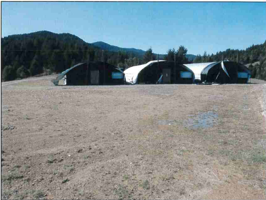
Photo 4. The preexisting cultivation infrastructure located in Area 1.
