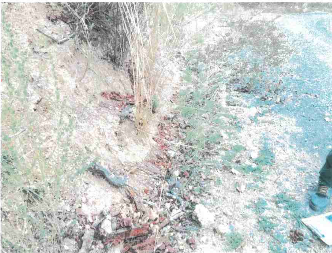
RP-6 Inside Ditch in Needs to be Cleaned
