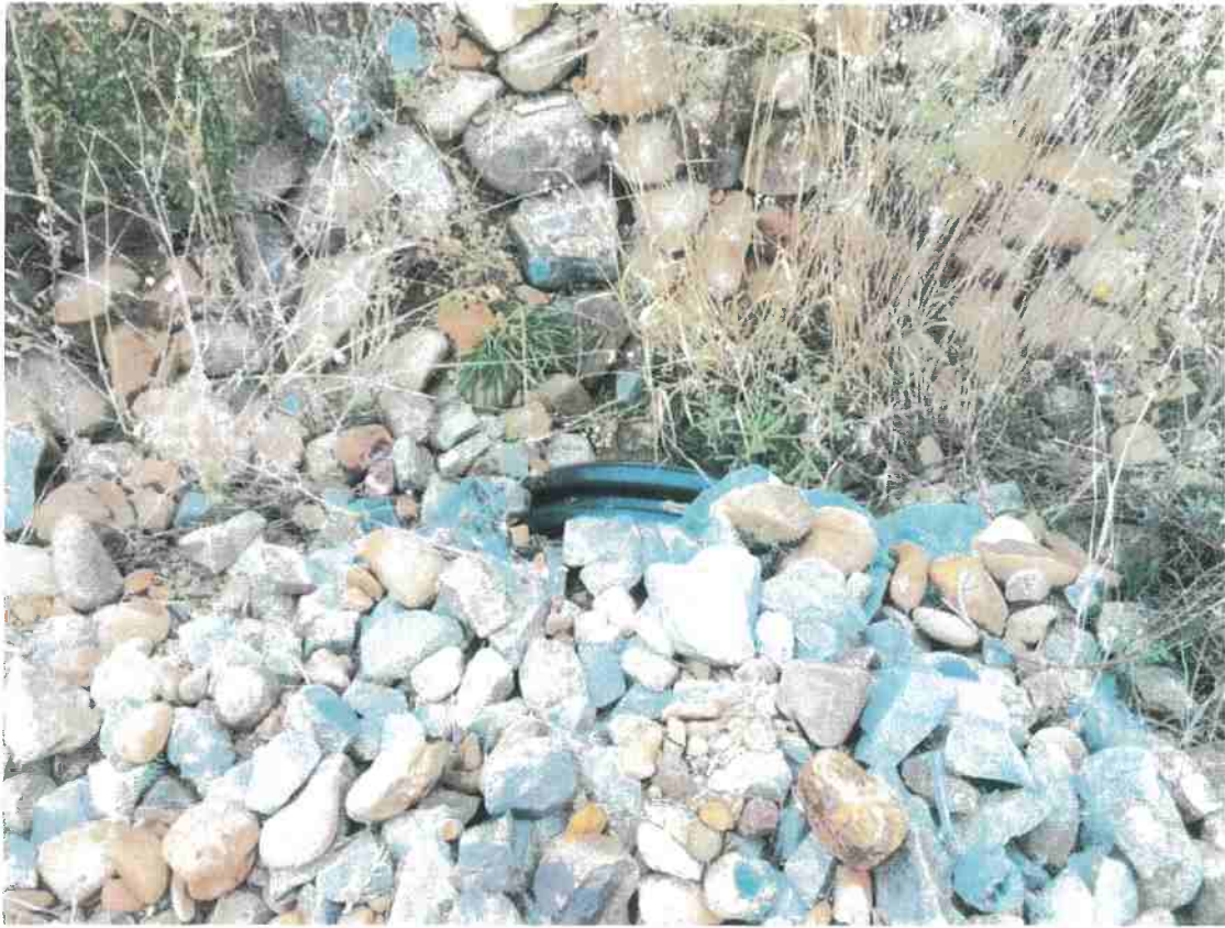
RP-7 Existing DRC Maintain Inlet to keep Clear of Debris.
