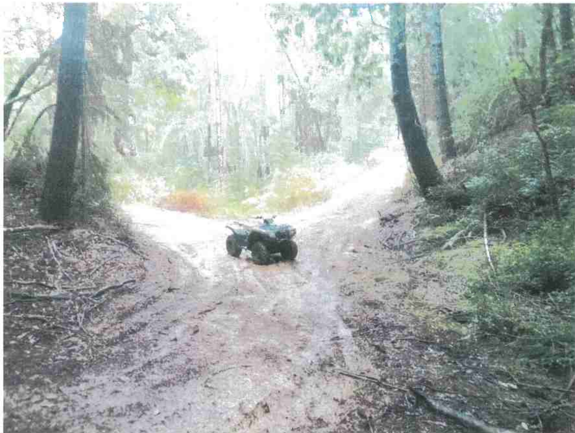
RP-34: Class III Stream Crossing with no Drainage Structure Install Culvert.
