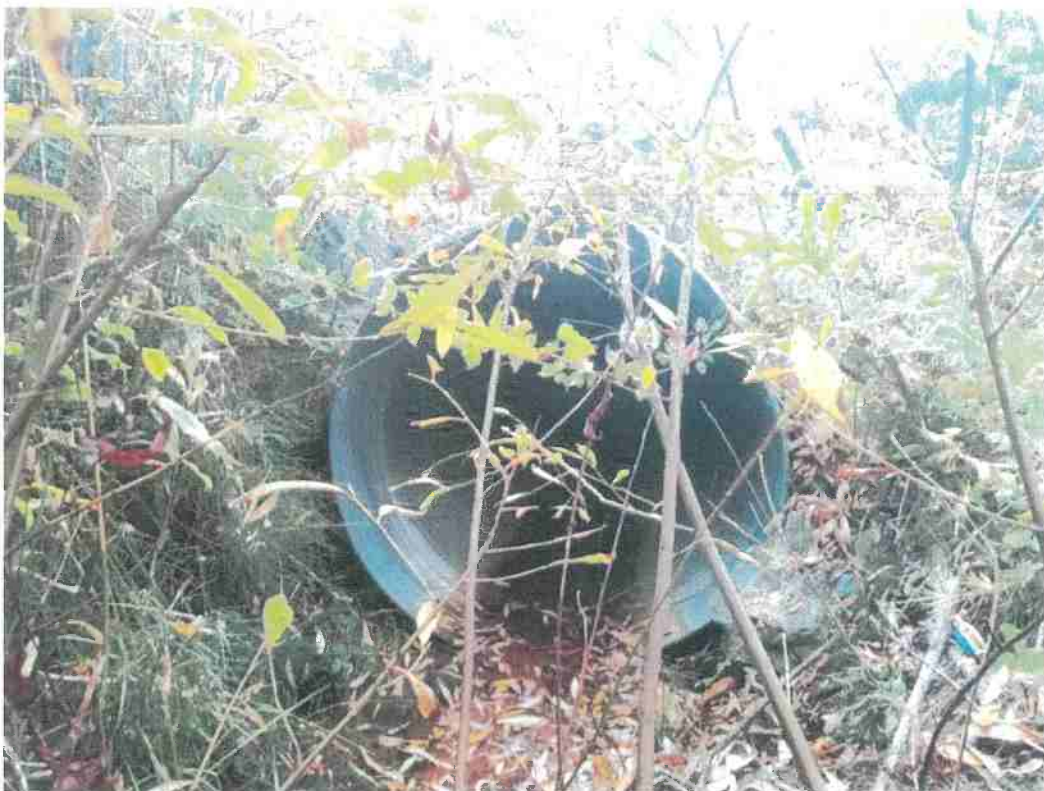
RP-1 Main Access Road: Class II Stream Crossing 54" Culvert.
