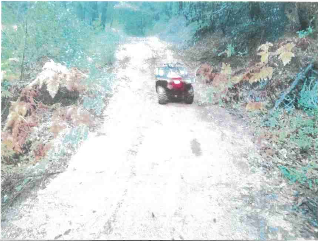
RP-32: Rock Existing Rolling Dip
