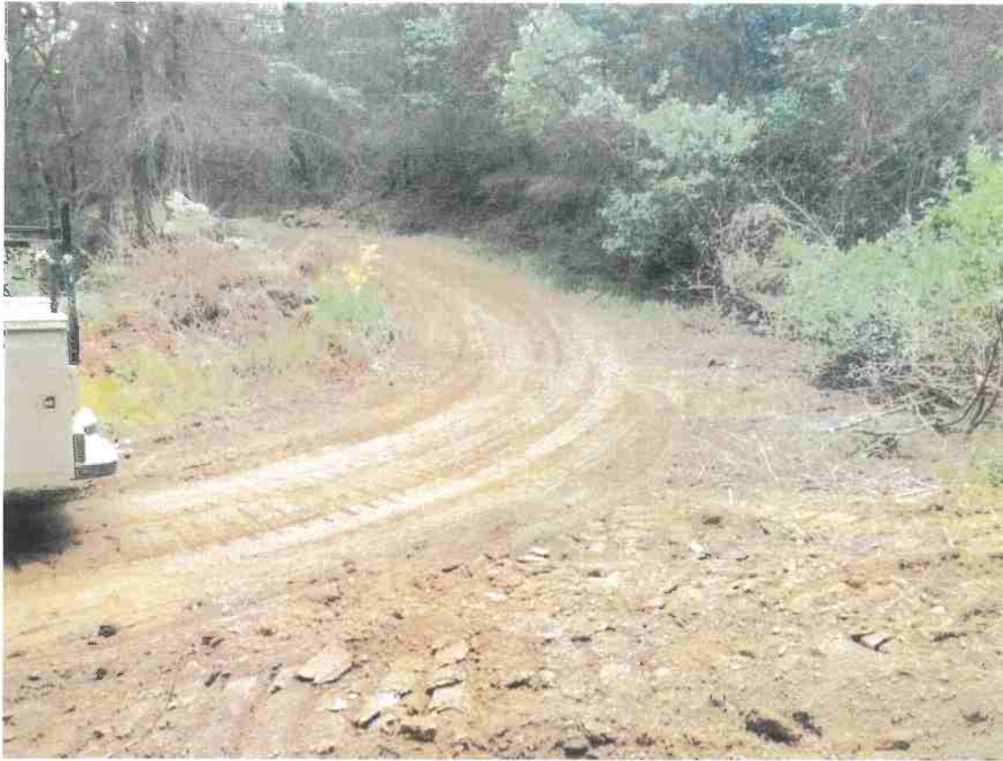
RP-24: Install Rocked Rolling Dip and Rock Approaches Where Road Crosses Above Class III Stream
