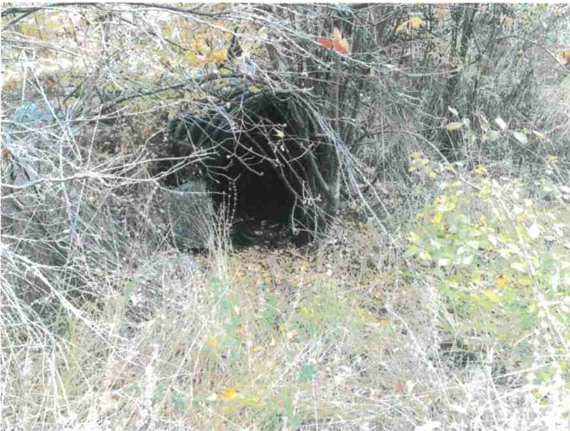
RP-8 Main Access Road: Class III Stream Crossing 36" Culvert
