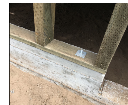
House bolted to foundation
